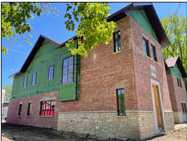
Photos taken of the construction progress in mid-June (Brandon Wilsey)
