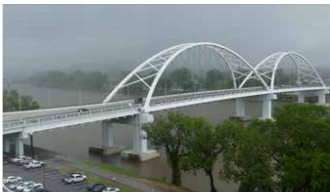
Bridge to Little Rock
