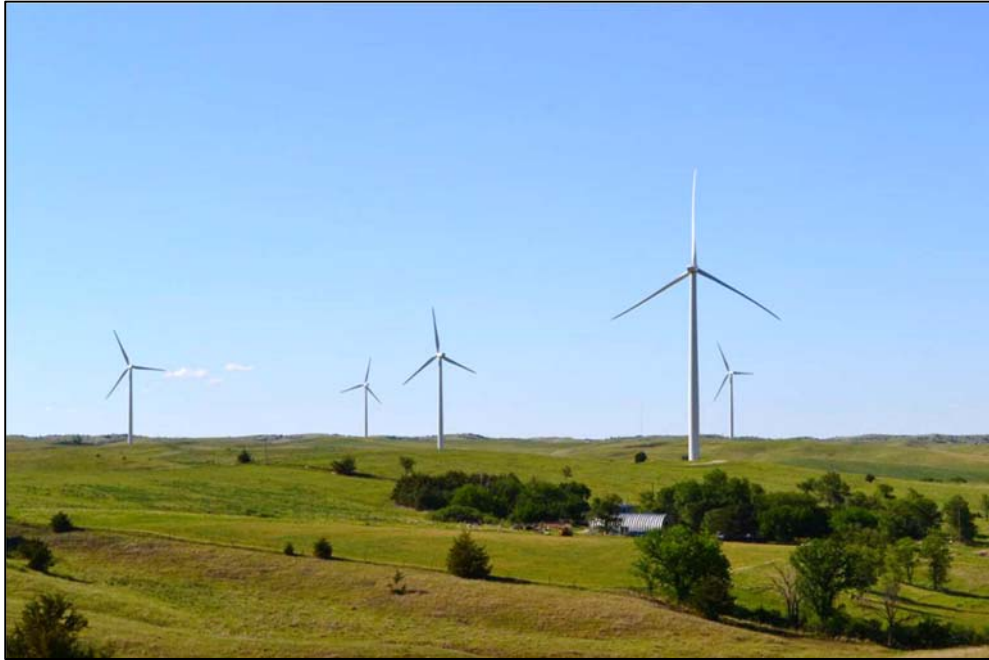
Broken Bow, Nebraska Wind Farm.
