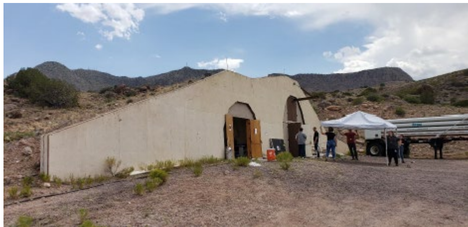
Figure 1. The "2-Ton" Bunker near Torres Laboratory
