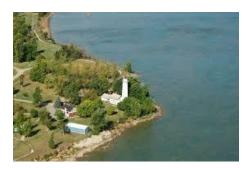
The Pointe aux Barques Lighthouse is one of the oldest lighthouses in Michigan. It remains in active service, with its light remotely controlled by the U.S. Coast Guard. The original lighthouse was built in 1848; due to problems in design and materials, the tower was rebuilt nine years later, in 1857. This structure, a cylindrical brick
