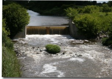
Drop Structure Before
