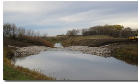
Drop Structure After
