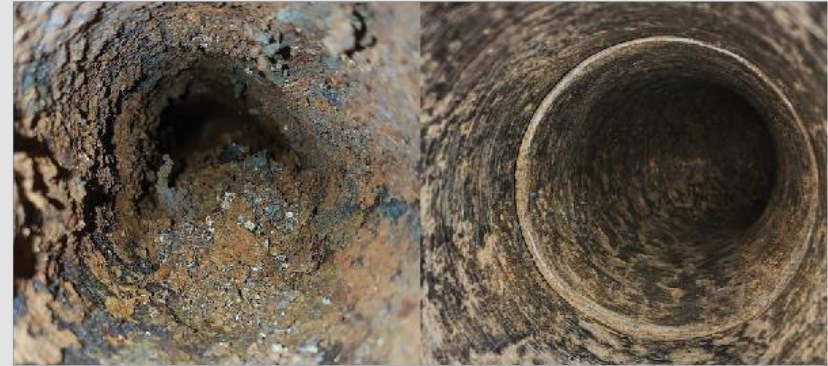
Descale rust buildup inside cast iron pipes.
