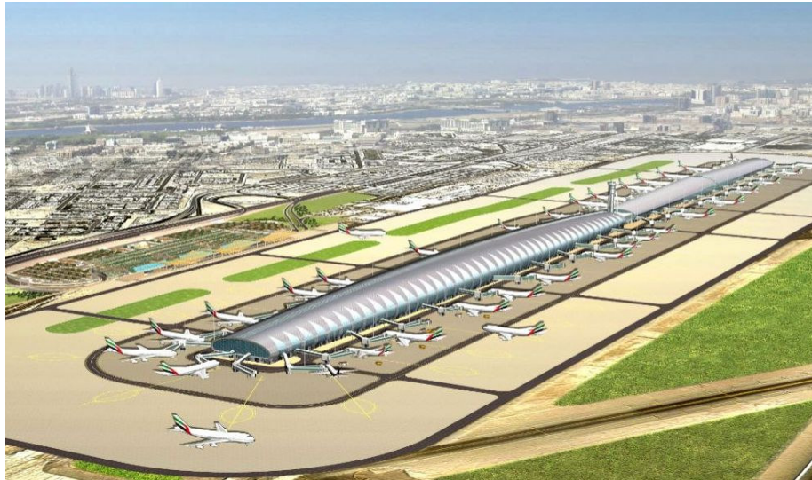
Figure 3-7: Dubai International Airport (Courtesy: Government of Dubai, Department of Civil Aviation)
