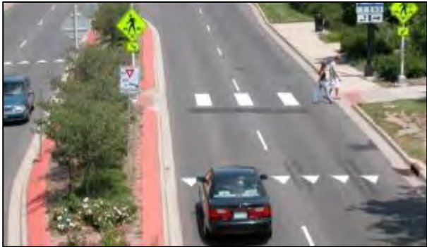
Advance yield stop lines and “shark teeth” make pedestrian crossings safer.
