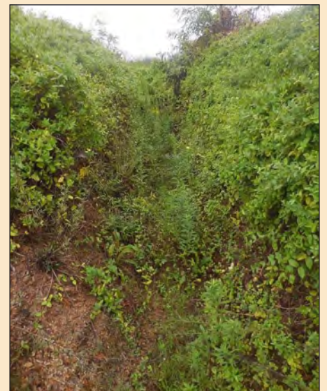
Commo trench at Newville
