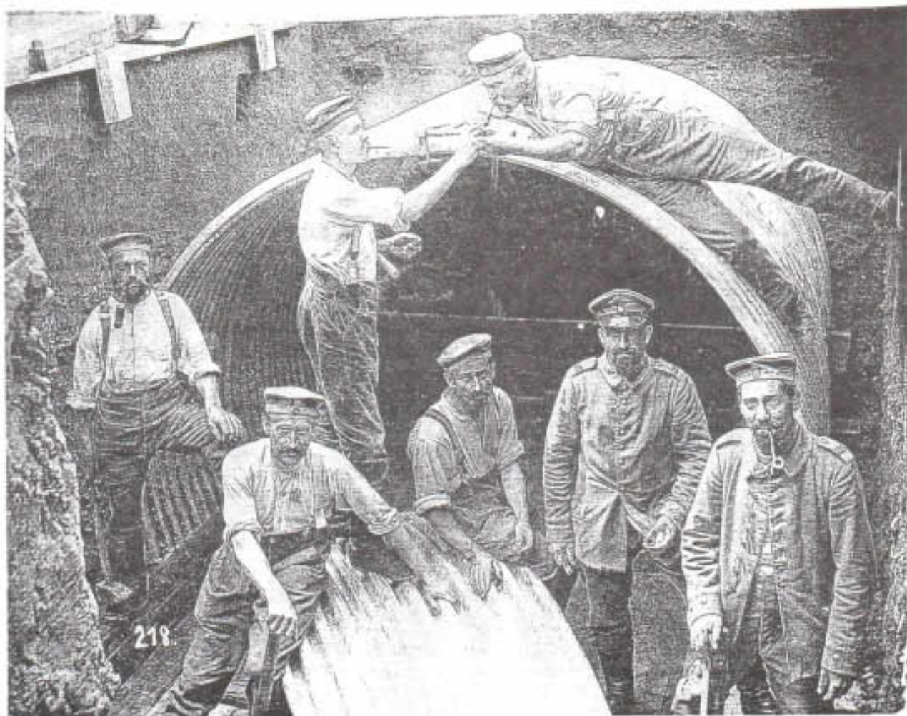
German shell-proof bunker under construction. Machine Guns and crews weathered artillery attacks in shell-proofs like this and emerged to set-up their guns in temporary positions when shelling stopped.
