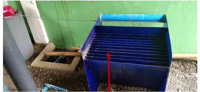
LAMELLA PLATES FOR CLARIFIER
