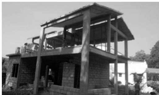
Figure 8: Villa under construction
