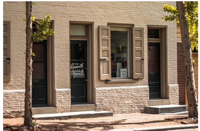
Courtesy of the Demuth Foundation
