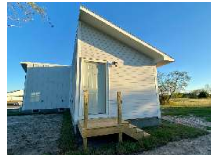
Completed MiCASiTA home in the RGV, back
