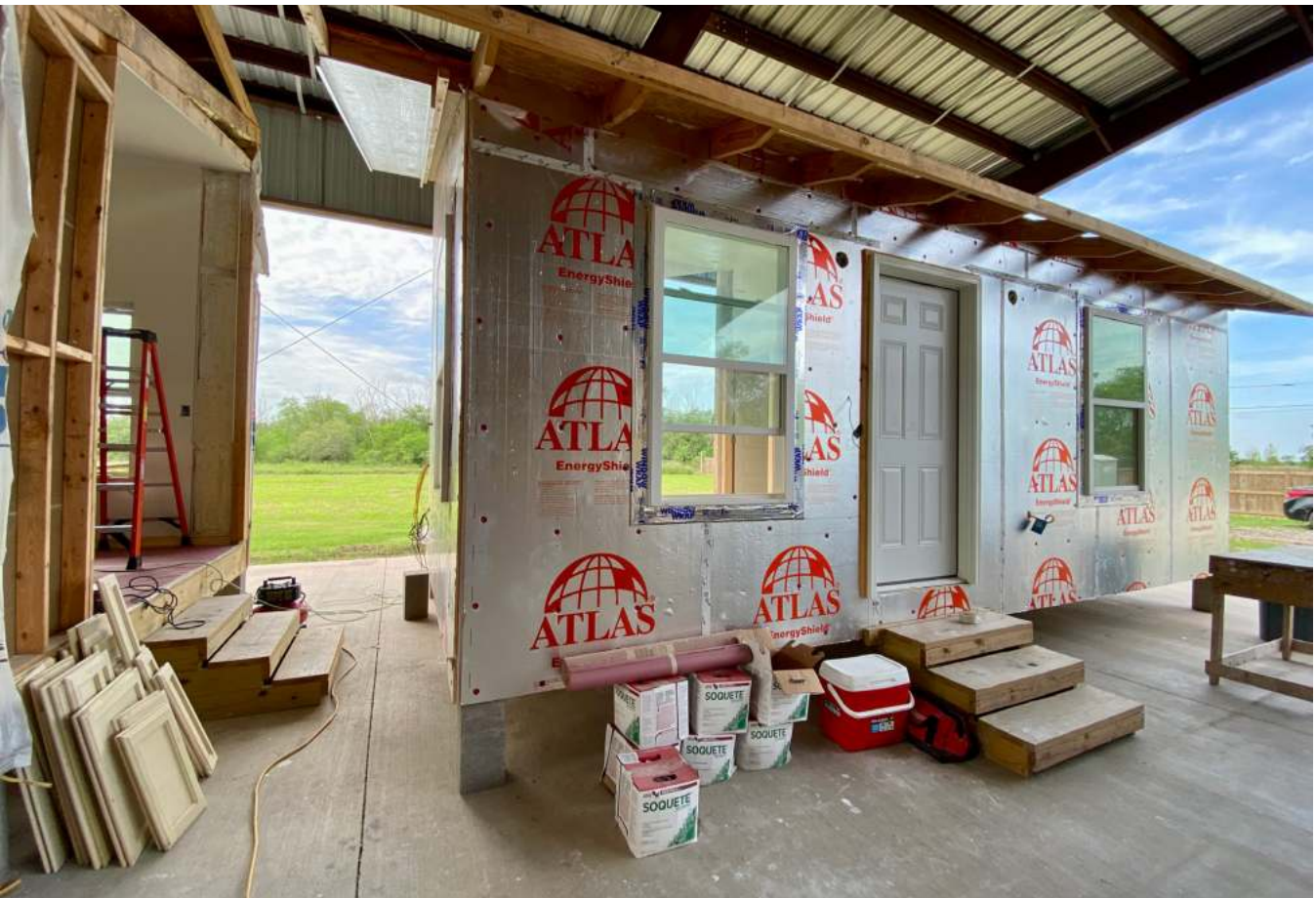
The factory requires both work stations for the boxes, and space to lay out and assemble large amounts of material.
