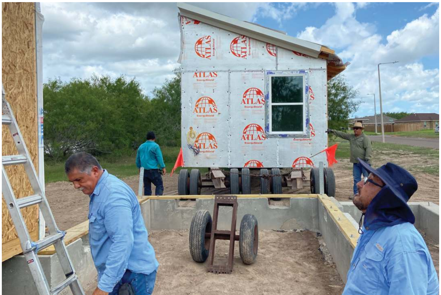
Boxes being moved from the truck to the foundation on site
