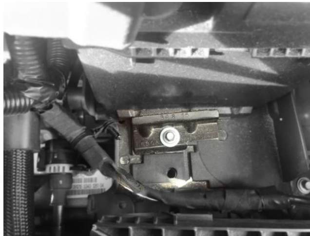
Figure 4: Battery tie down and hole to be drilled out
