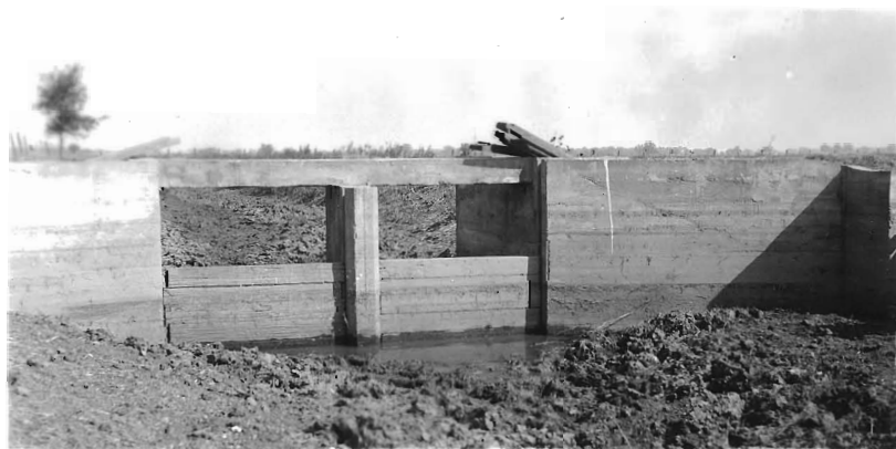
Fig. 8 - Acacia Canal - Combined Check and Delivery Gate - September 23, 1936
