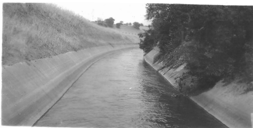
Fig. 10 - Adams Canal, Concrete Lined Section 500 Feet Below Intake - September 23, 1936
