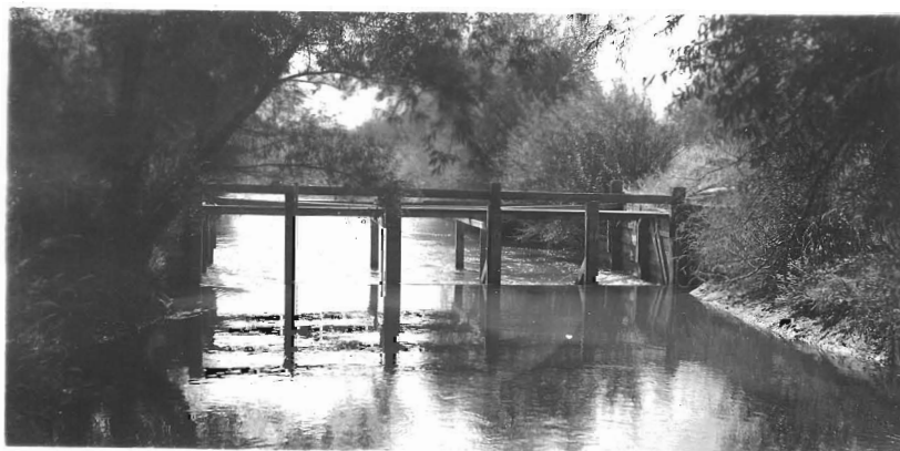
Fig. 12 - Winters Canal, Unlined Section, Timber Check Gate and Drop - September 23, 1936
