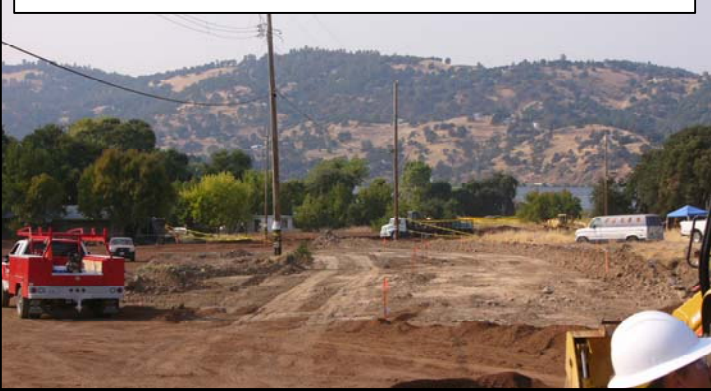
Photo taken 9-14-06 of eastern edge of graded area showing depth of cut below ground surface.
