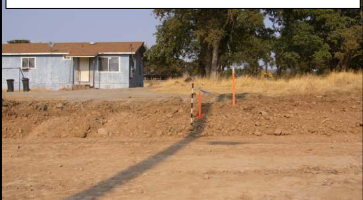
Photo taken 9-14-06 of eastern edge of graded area showing depth of cut below ground surface.
