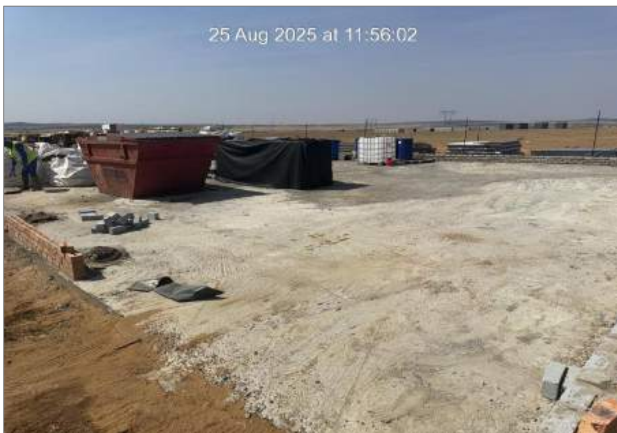
Figure 6: Bundled waste area
