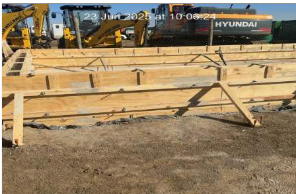
Figure 4: Diesel and Chemical bund under construction
