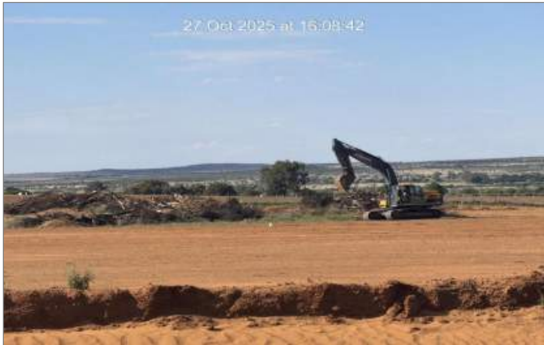
Figure 5: Cleared vegetation being moved from site.
