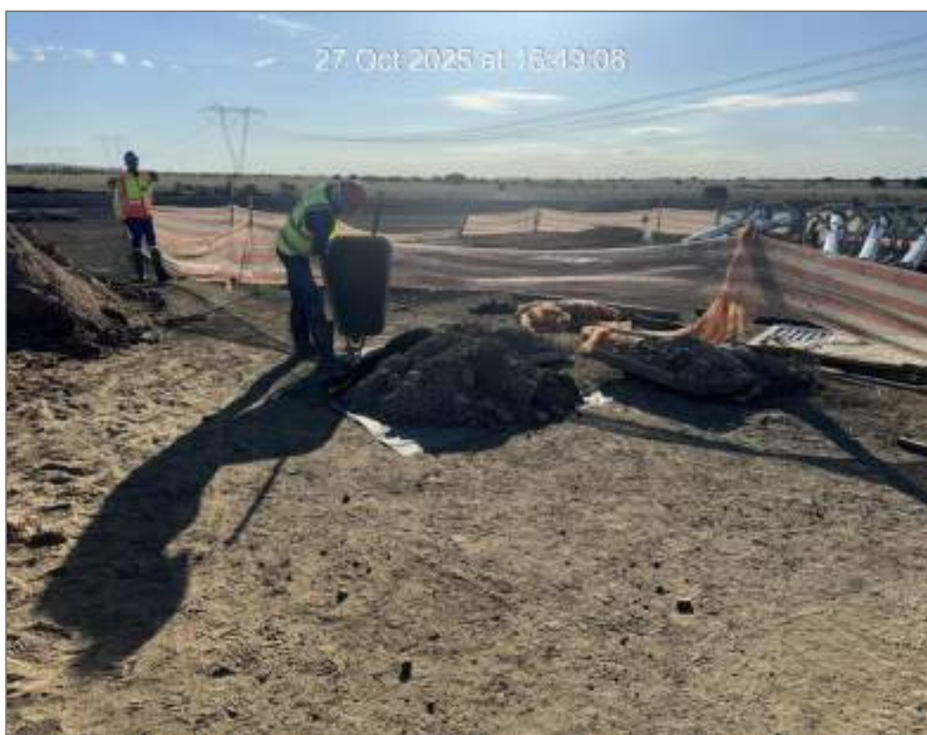
Figure 10: Concrete being placed on plastic bags.
