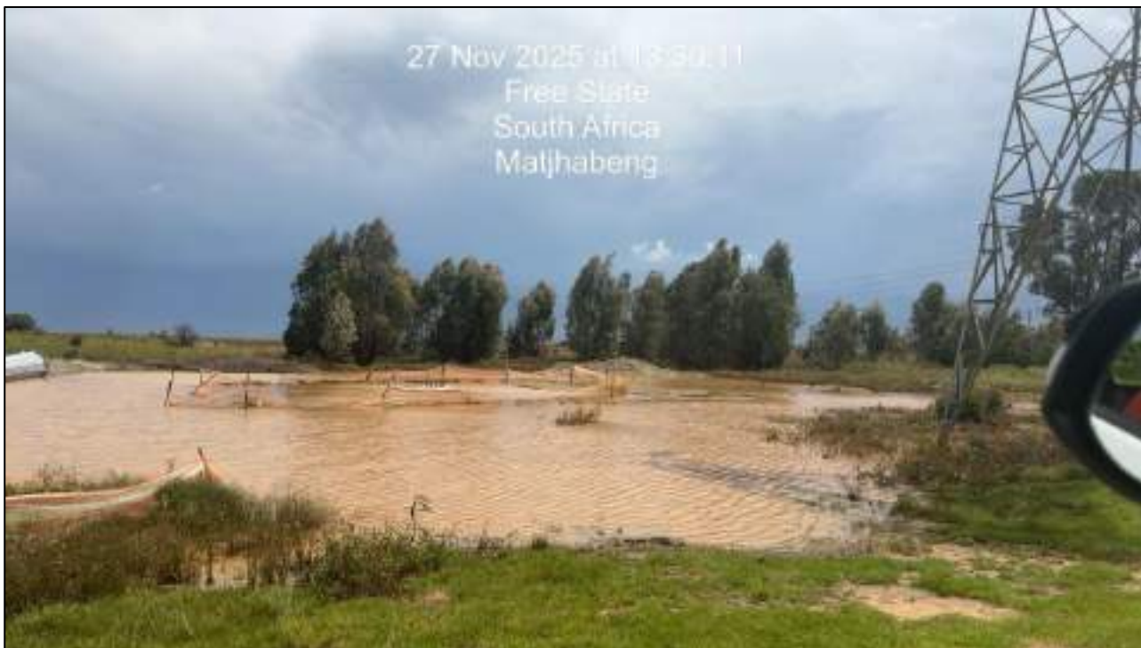
Figure 3: Rainwater accumulated at Tower No. 13
