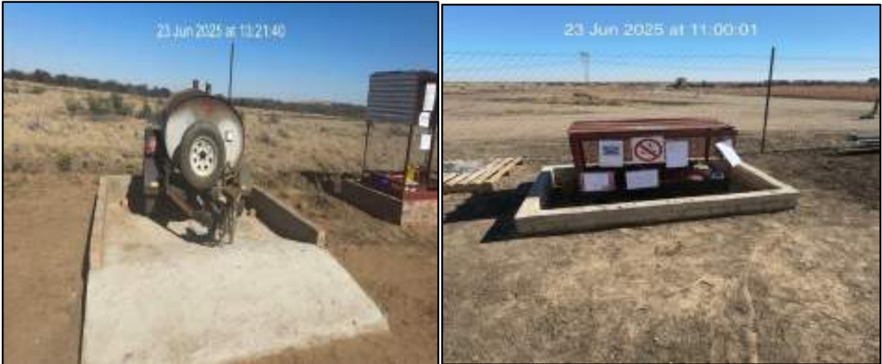
Figure 5: Diesel buzzer on an impervious surface and hazardous chemical bund.
