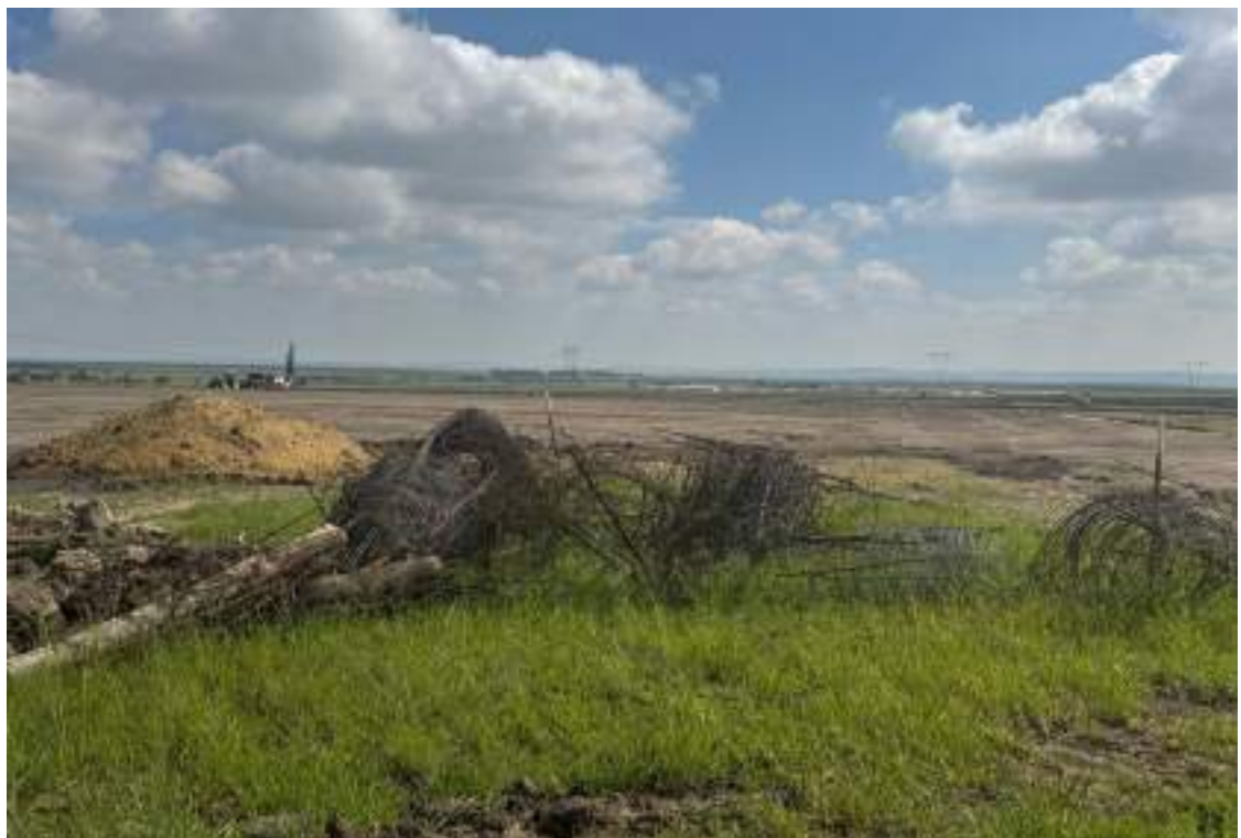
Figure 2: Removed fences must be reused or appropriately disposed of.
