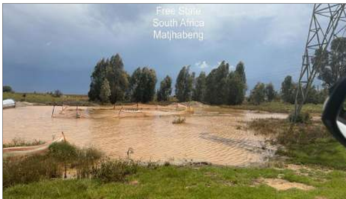
Figure 3: Rainwater accumulated at Tower No. 13
