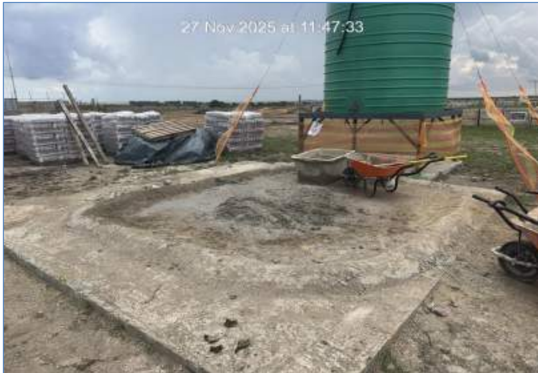
Figure 9: Concrete slab for concrete mixing
