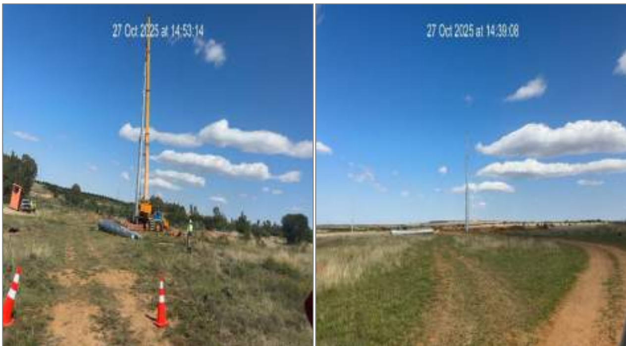
Figure 5: Erected Monopole Tower.
