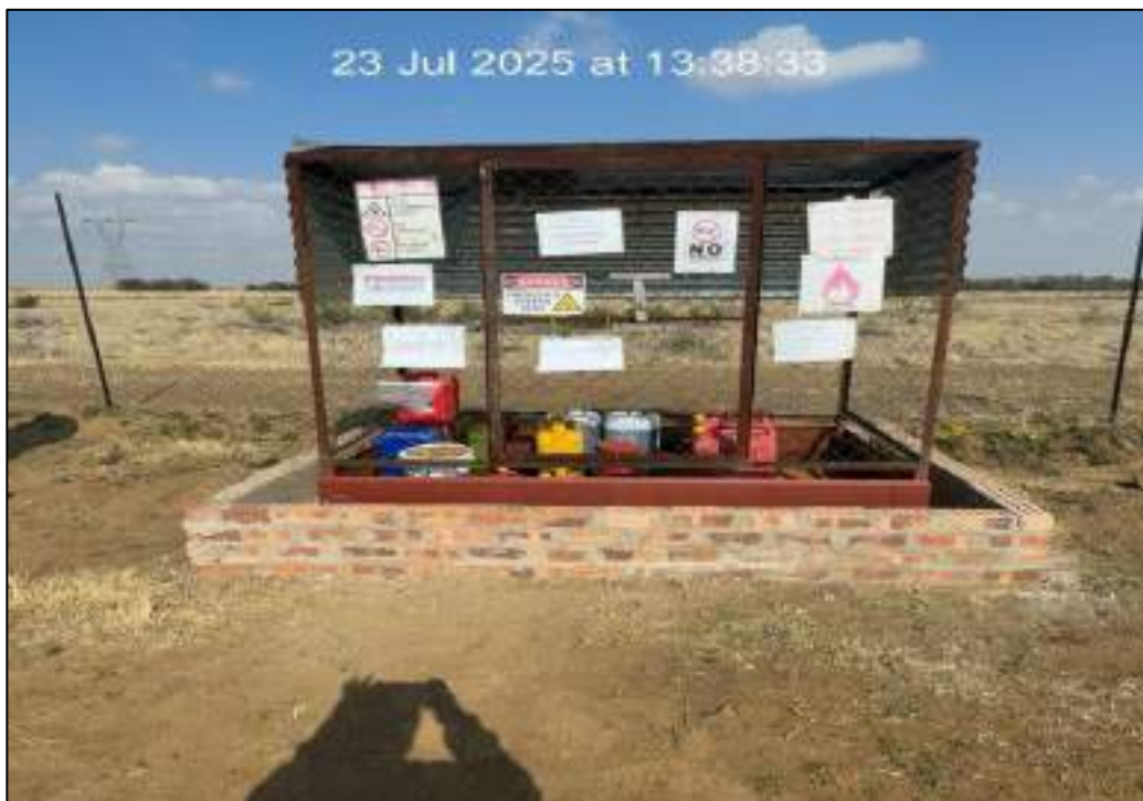
Figure 4: Bund and roofed chemical storage area.
