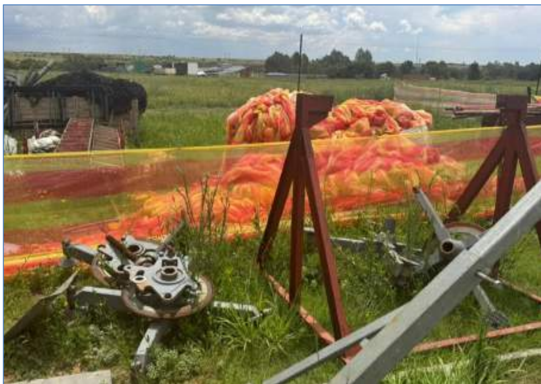
Figure 8: Torn barricading nets must be taken for recycling.
