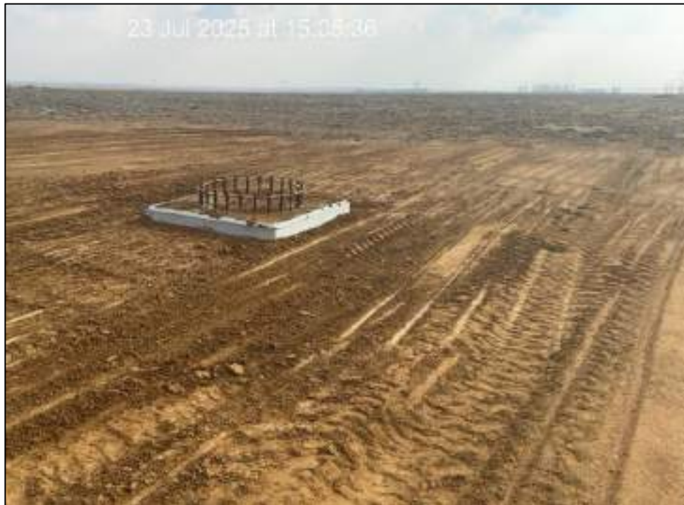
Figure 7: Filled in pits where topsoil must only be spread after completion of structures
