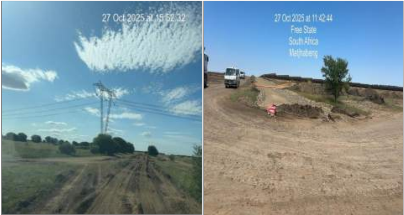
Figure 7: Poor condition of the access roads
