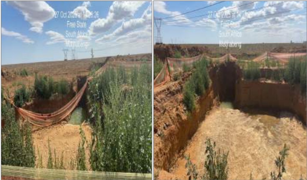
Figure 7: Groundwater encountered.
