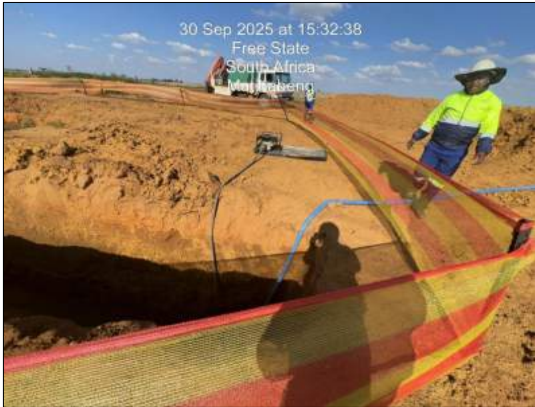
Figure 5: Groundwater being pumped out of excavations.
