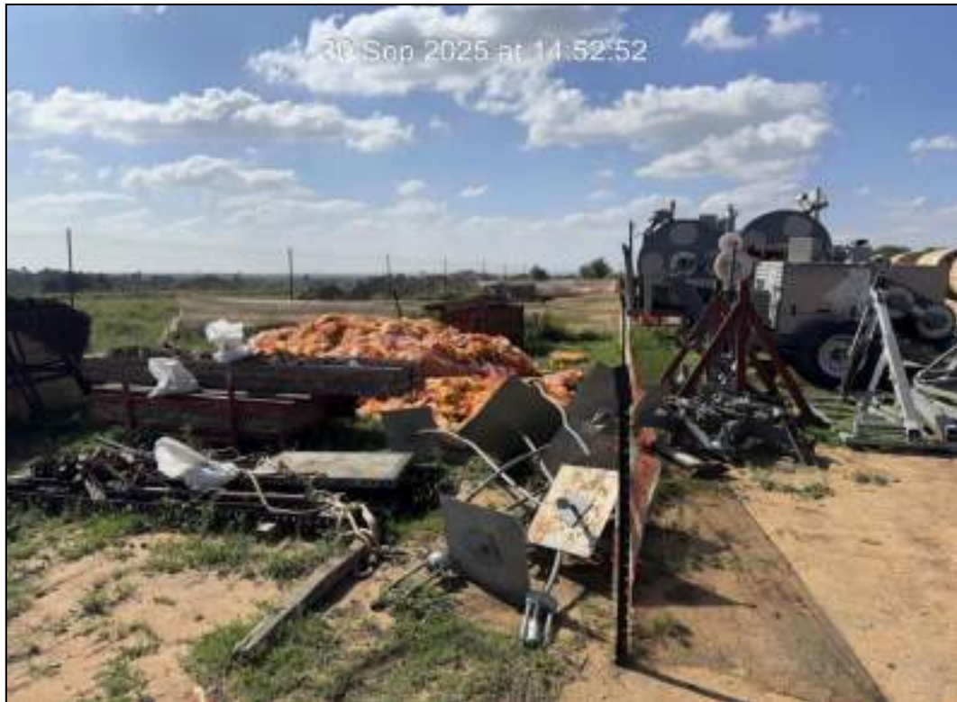
Figure 3: Torn barricade must be recycled.
