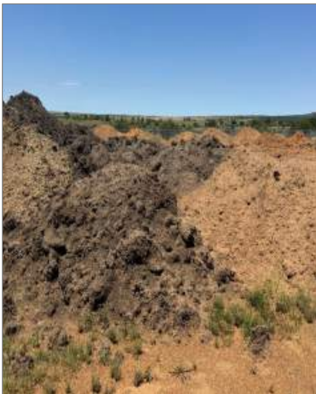
Figure 6: Topsoil being mixed with subsoil
