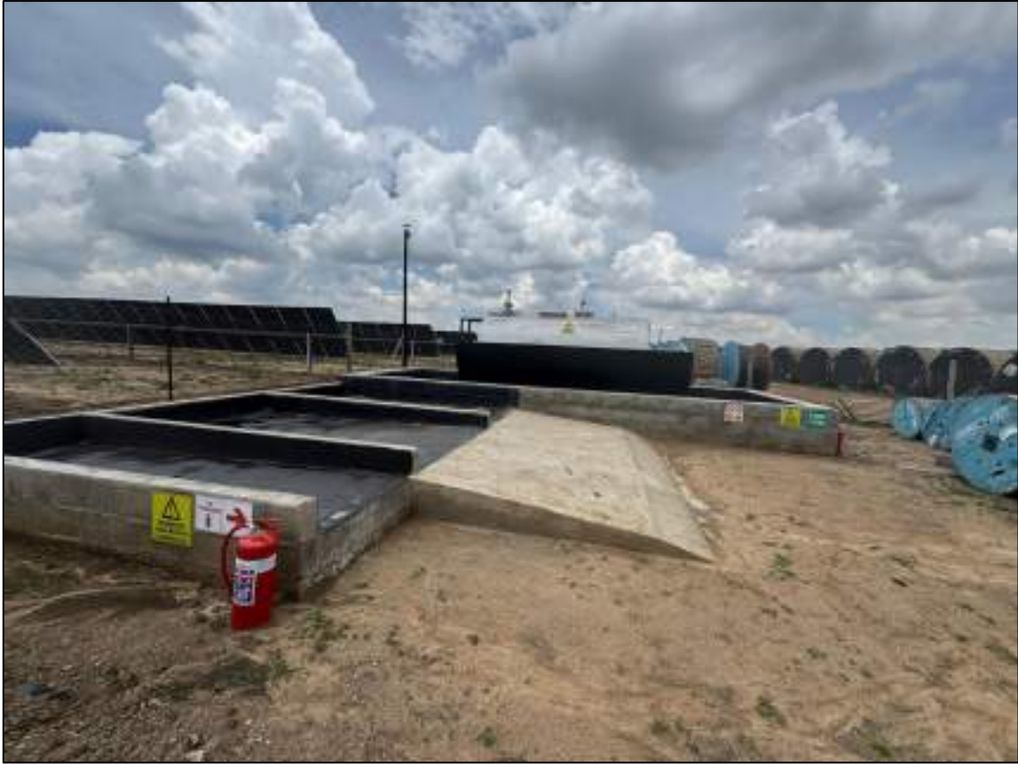
Figure 11: Newly constructed diesel bund.
