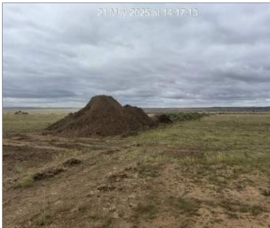
Figure 2: Stockpile exceeding 2m in height.
