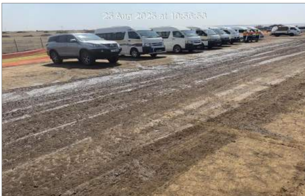
Figure 2: Nuisance due to water from the bowser
