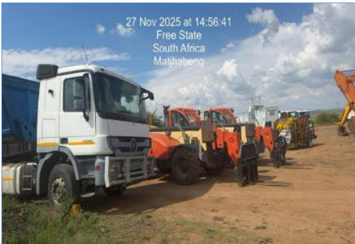
Figure 8: Machinery standing without drip trays
