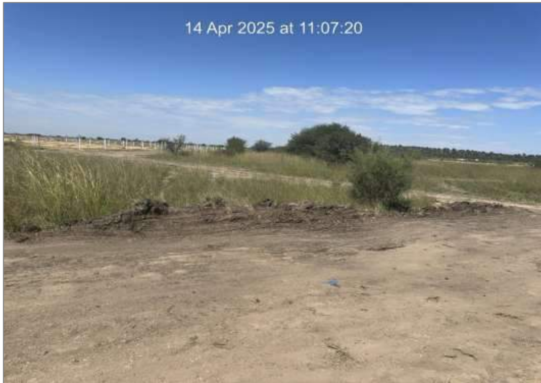
Figure 3: Roads requiring regrading
