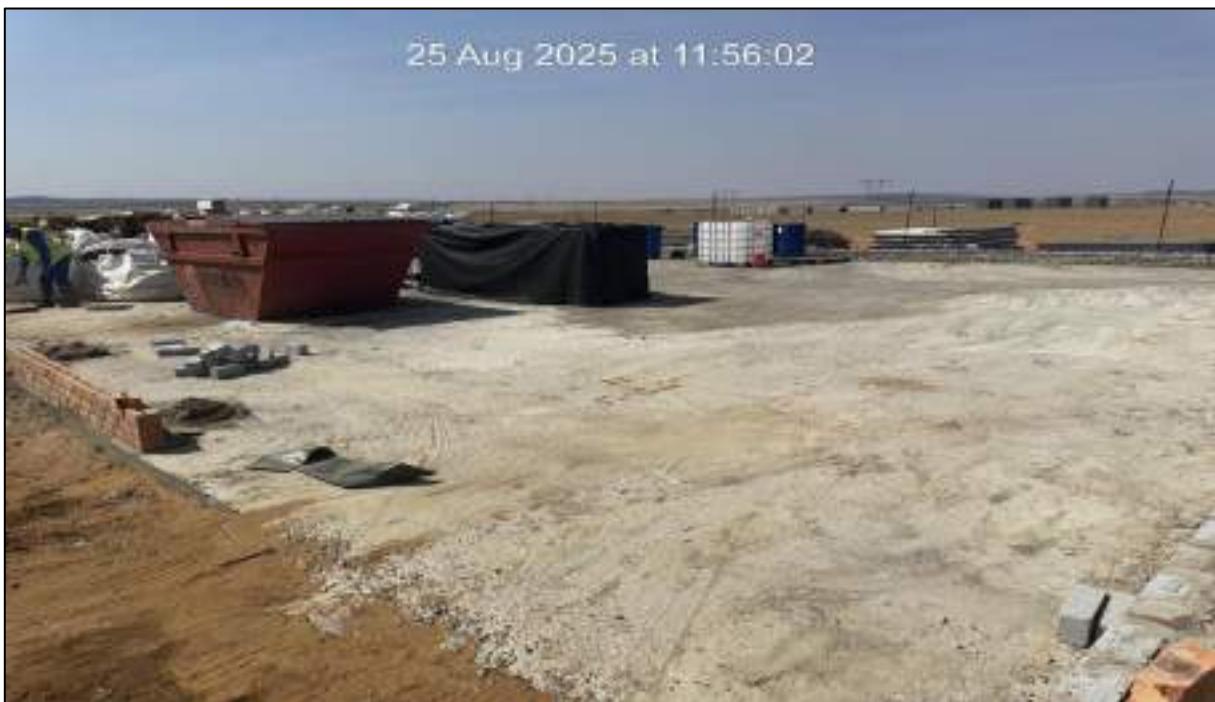
Figure 8: Waste bund construction in place
