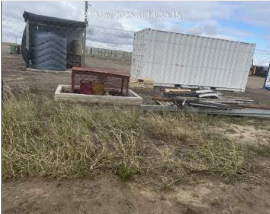
Figure 1: Chemical bund onsite.
