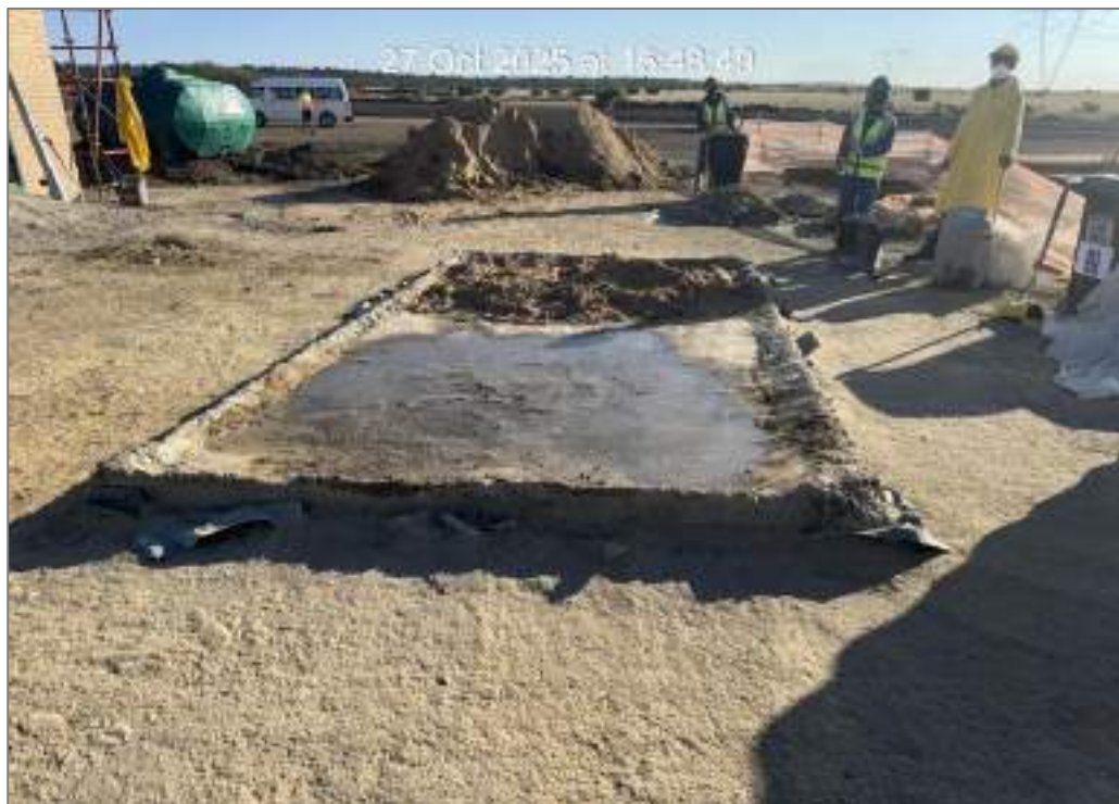
Figure 9: concrete being mixed on a concrete slab.
