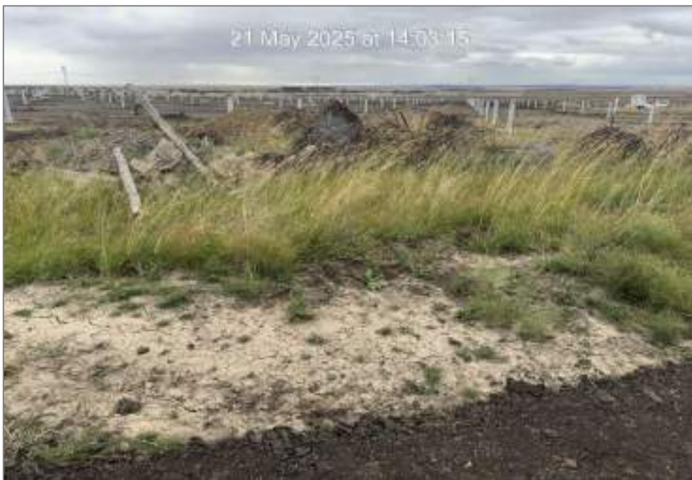
Figure 4: Old fences that must be removed.
