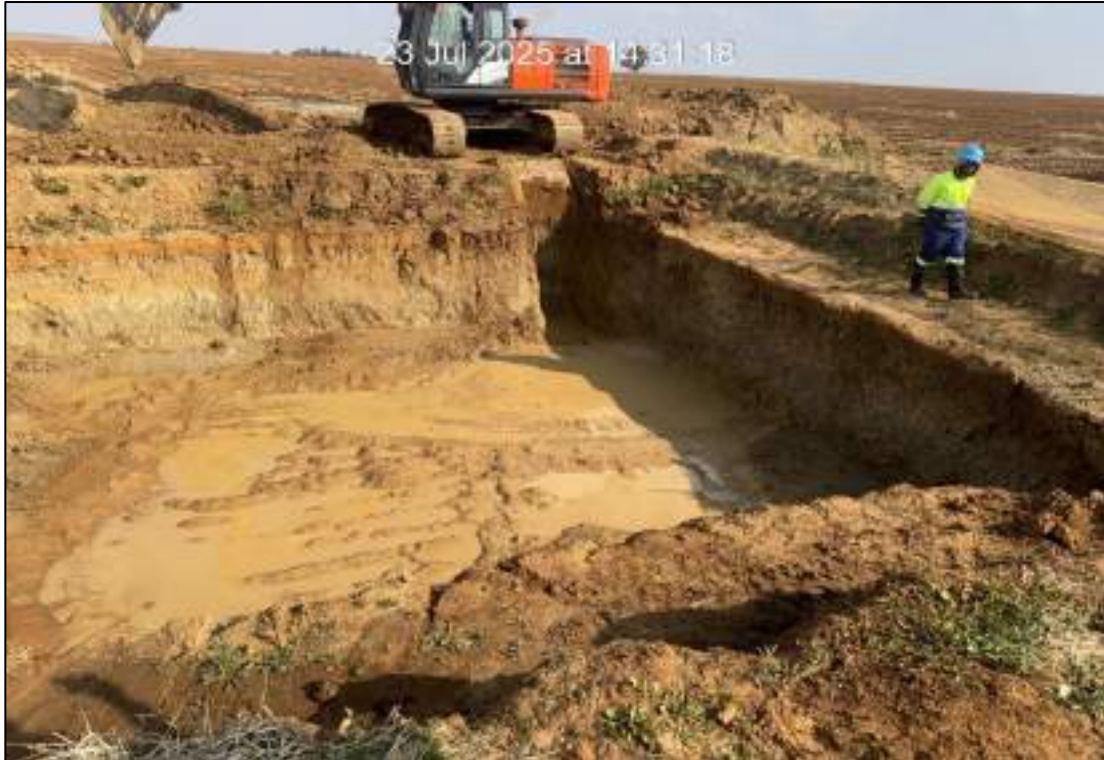
Figure 6: Groundwater that must be pumped out before concrete is poured.
