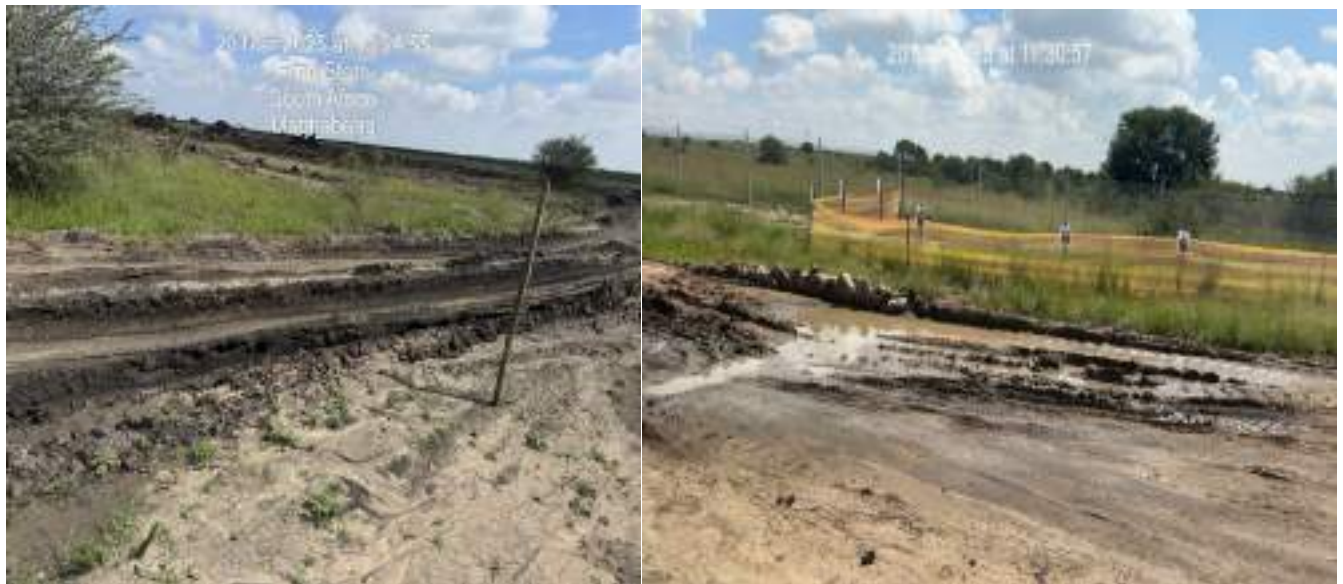
Figure 4: Roads requiring regrading
