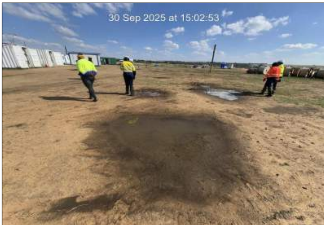
Figure 4: Water ponding on the laydown area.
