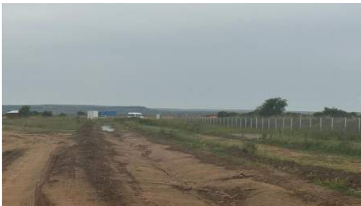
Figure 5: Constructed stormwater berms
