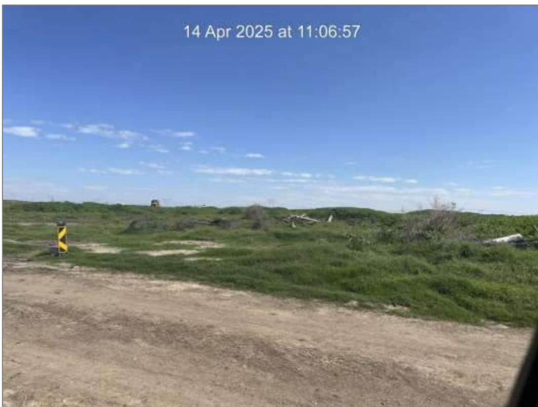
Figure 2: Removed fences must be reused or appropriately disposed of.
