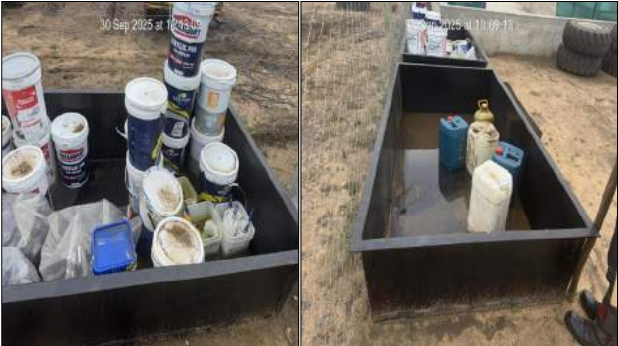
Figure 7: Chemical bund accumulating rainwater.
