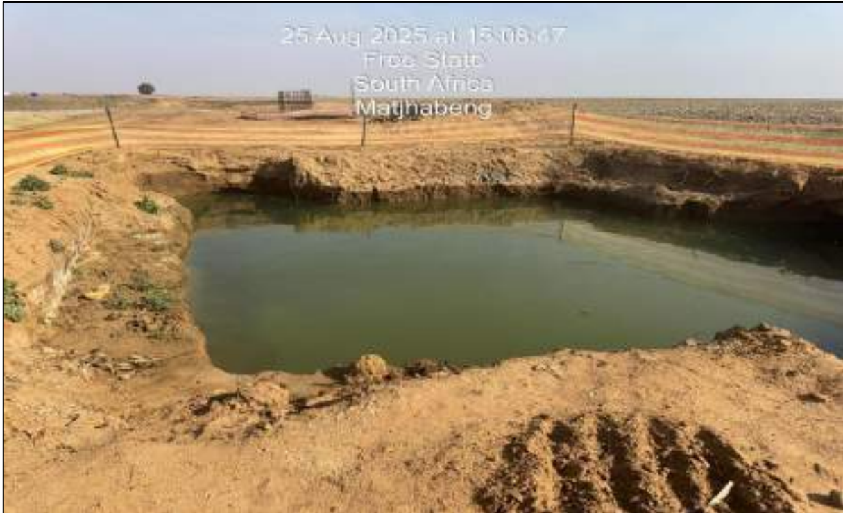
Figure 1: Groundwater encounter on some of the pits.
