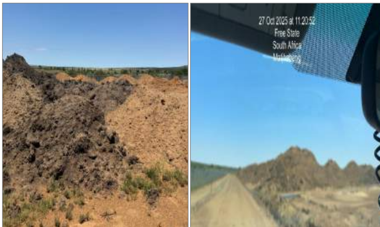
Figure 12: Stockpile height exceeding 2m.
