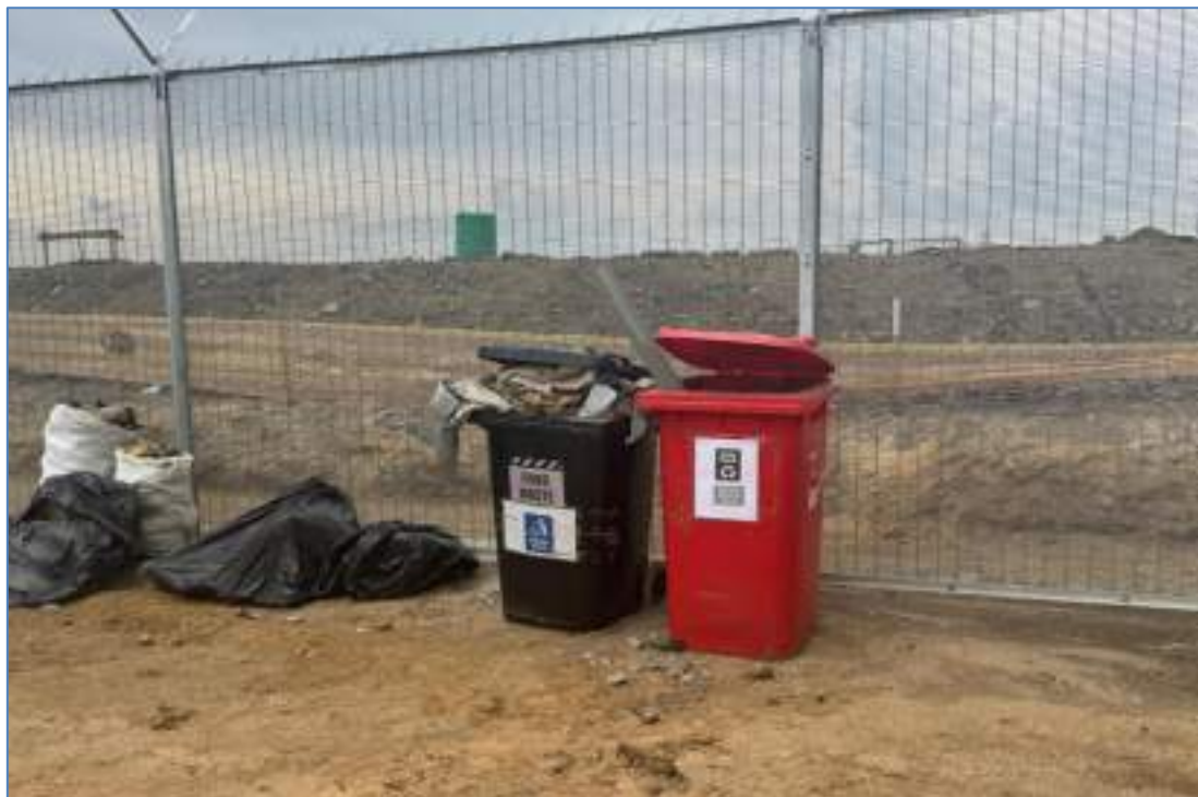
Figure 6: Bins overflowing with waste at the switching station
