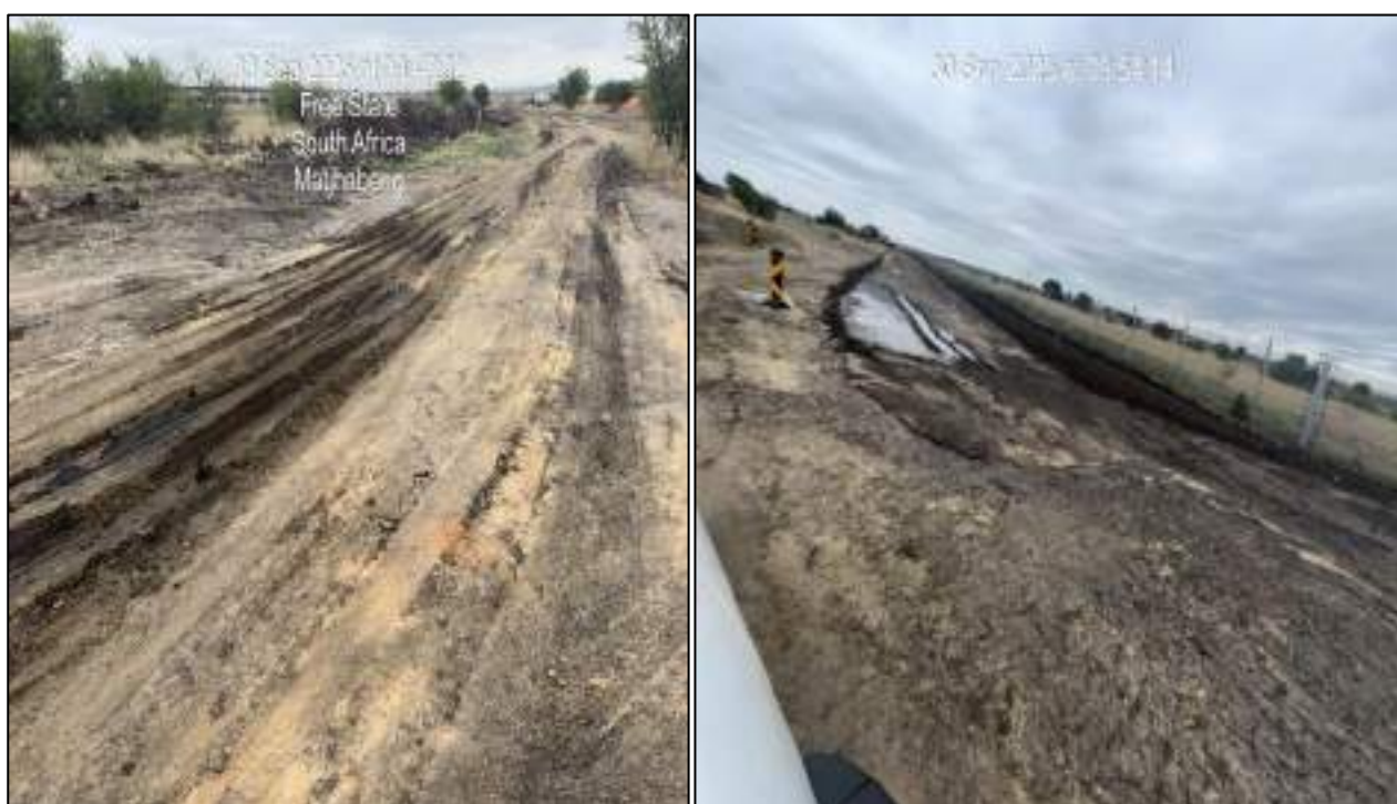
Figure 10: Condition of the access road.
