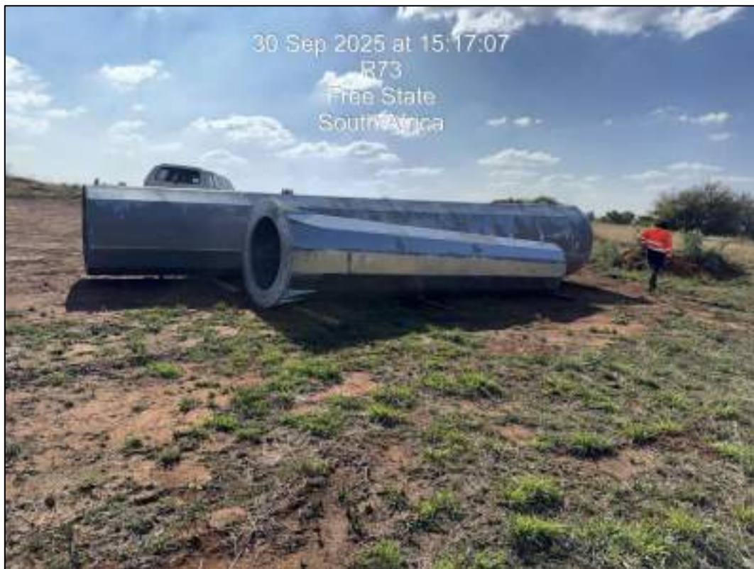
Figure 6: Pylons (material) onsite.
