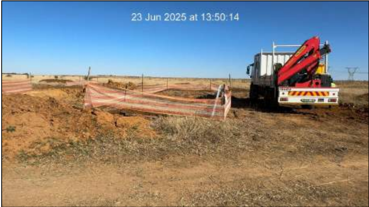
Figure 3: Barricaded excavation along the line.
