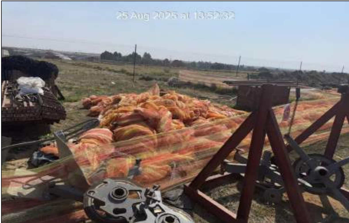
Figure 7: Stored barricade material to be used at the trenches.
