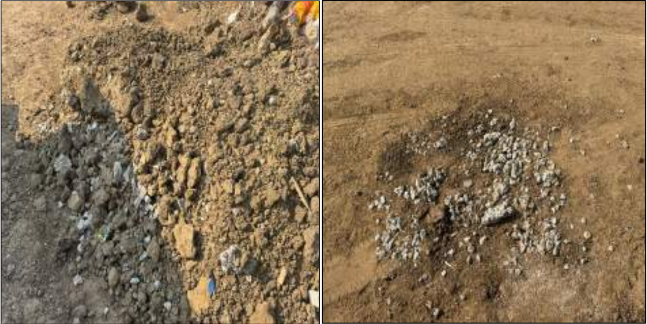
Figure 3: Concrete that must be removed from the construction area for disposal.
