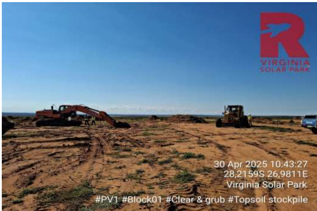
Figure 8: Ongoing alien vegetation clearance
