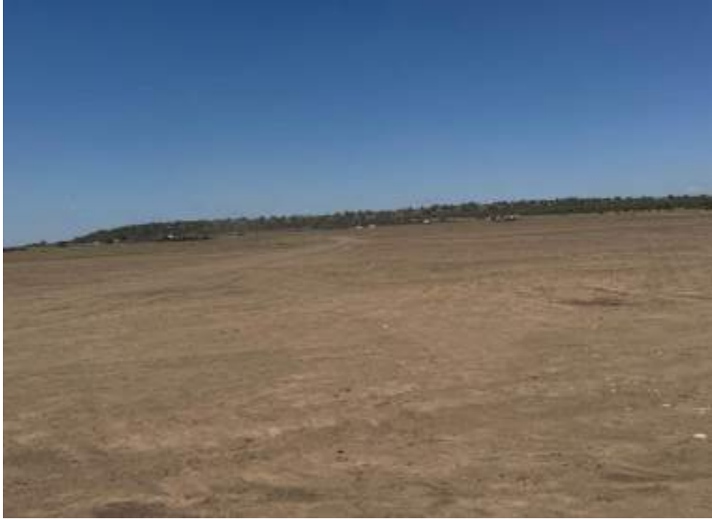
Figure 1: Extensive portion of the site that was cleared.
