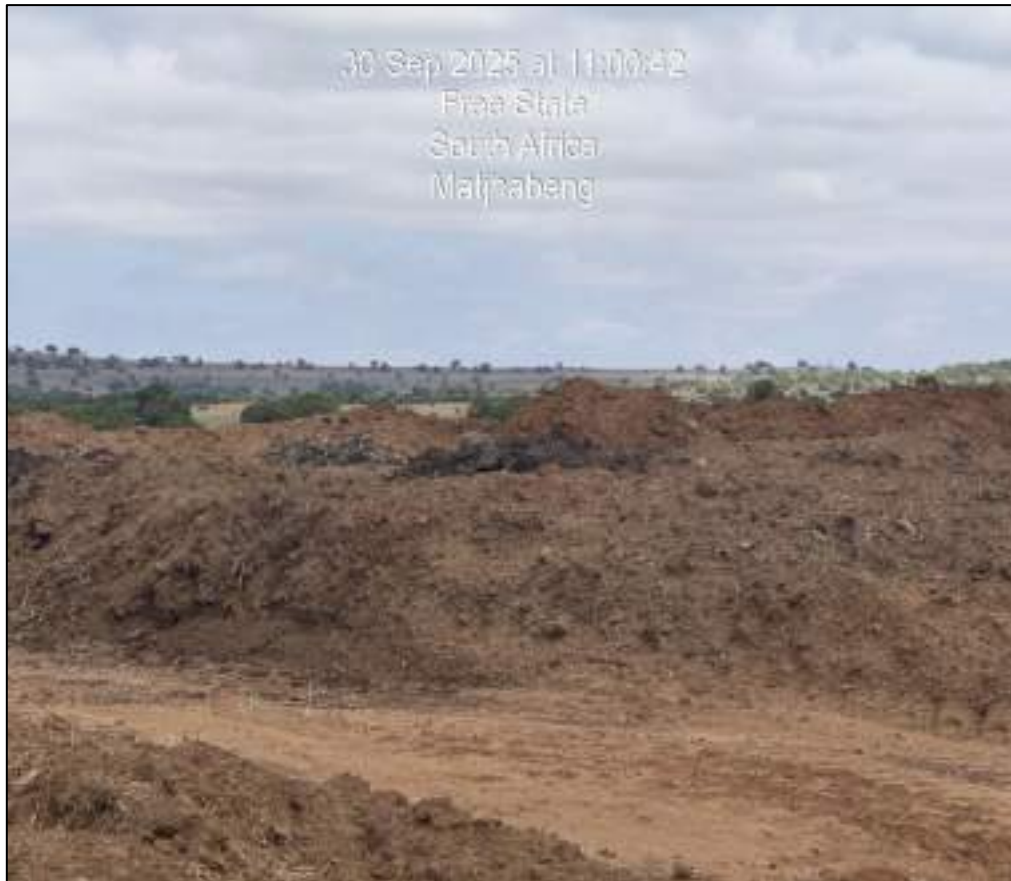
Figure 13: Topsoil mixed with spoil material.
