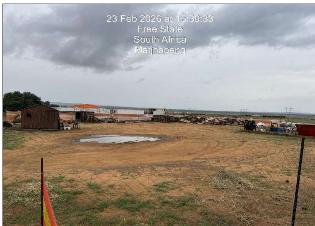
Figure 2: Water ponding at the waste area
