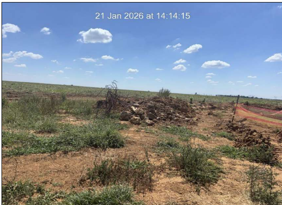
Figure 2: Rubble that must be removed from site.
