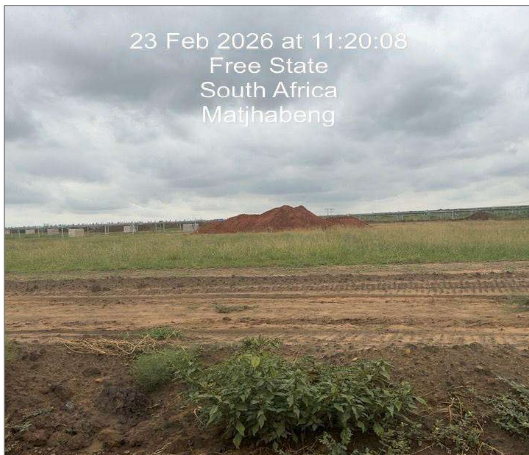
Figure 9: Stockpile height exceeding 2m
