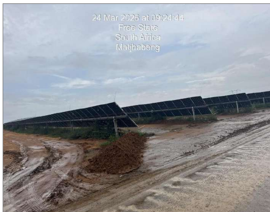
Figure 8: Erosion control measure
