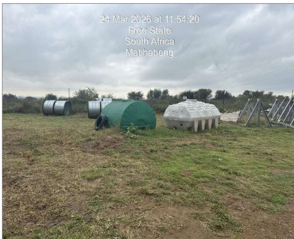
Figure 1: Cleaned section at the laydown area
