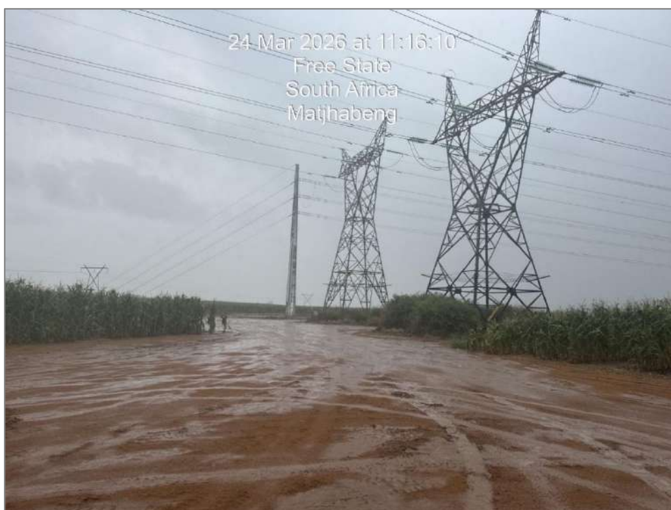
Figure 8: Stringing of the overhead powerlines
