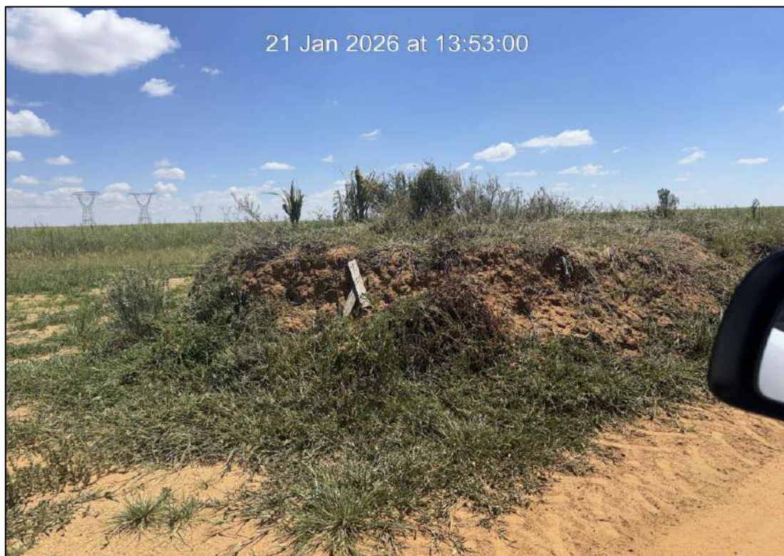
Figure 6: Topsoil stockpiles signs that must be replaced.
