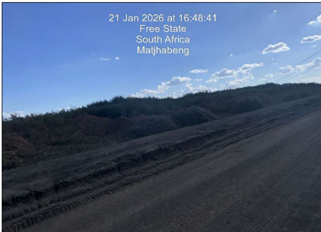
Figure 3: Cleared vegetation requiring to be disposed of.
