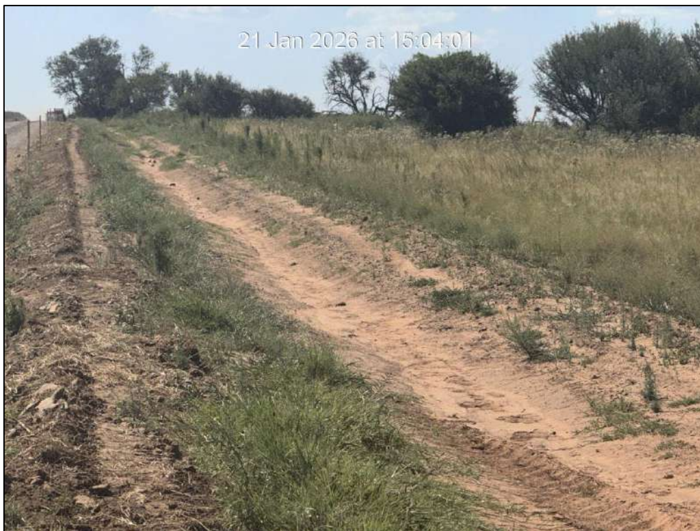
Figure 5: Constructed stormwater berms
