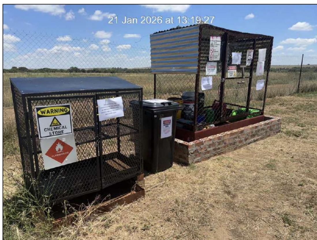
Figure 8: A new chemical bund.
