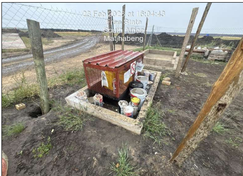
Figure 1: Chemical bund without a roof.
