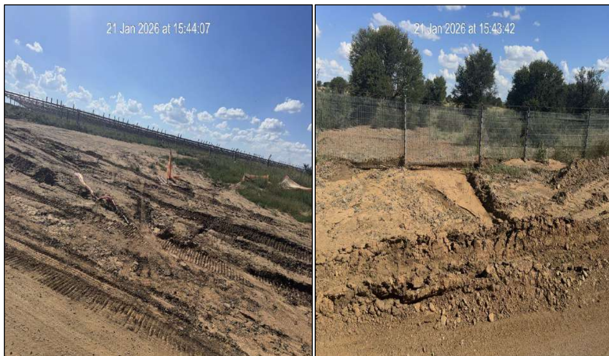
Figure 4: Erosion damage.
