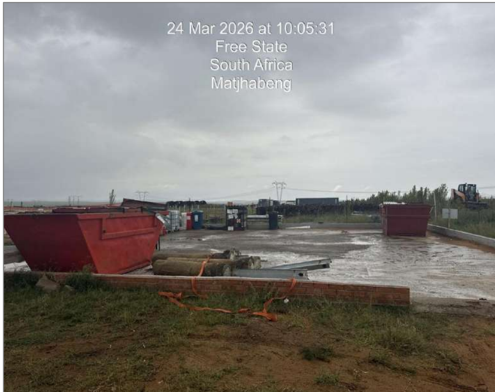
Figure 9: Clean waste area.
