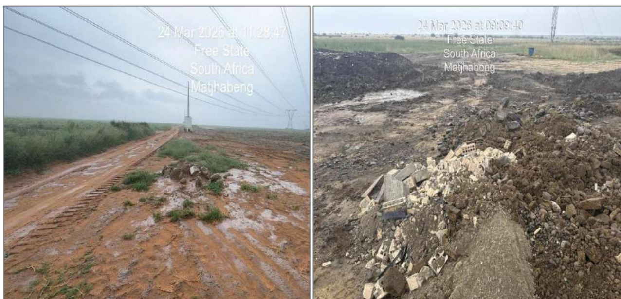
Figure 4: Construction Rubble on the line and switching station.
