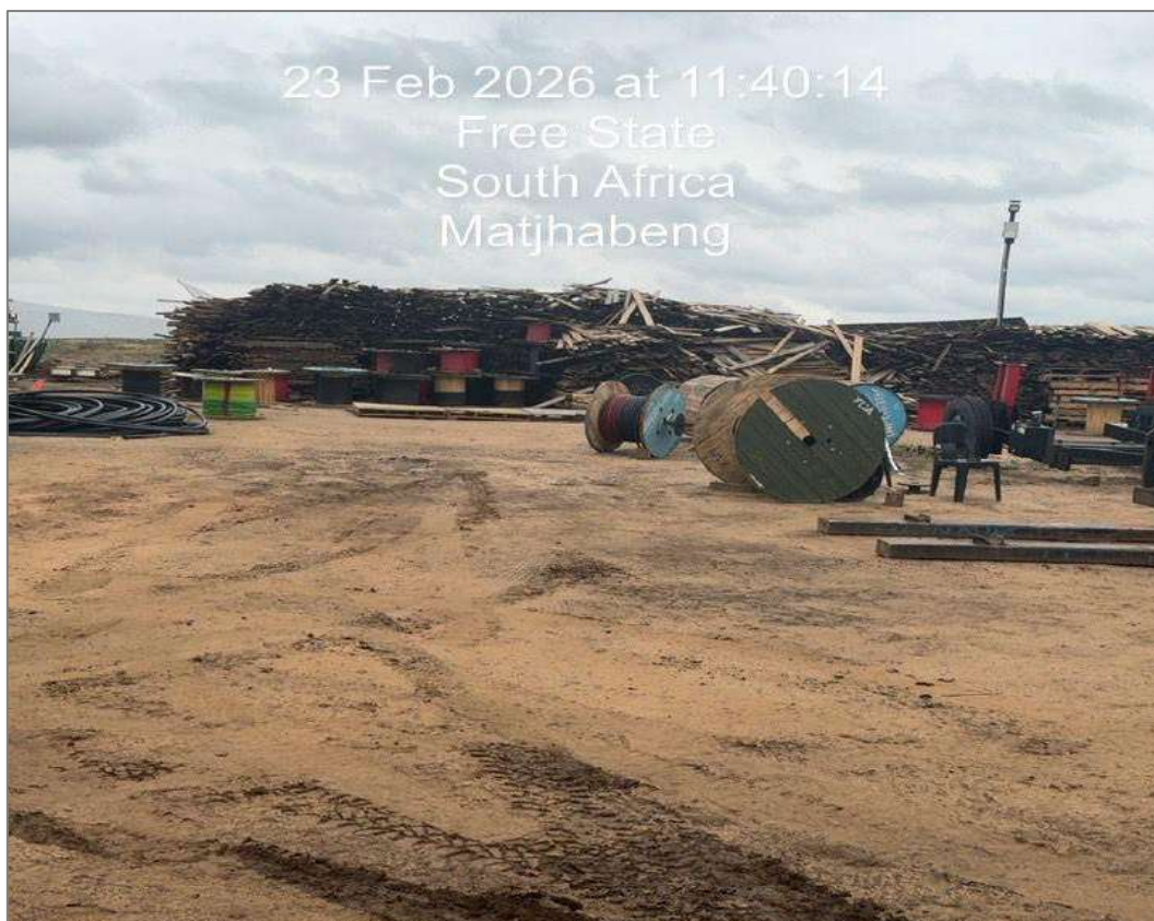
Figure 5: Large pile of wood that is a fire hazard
