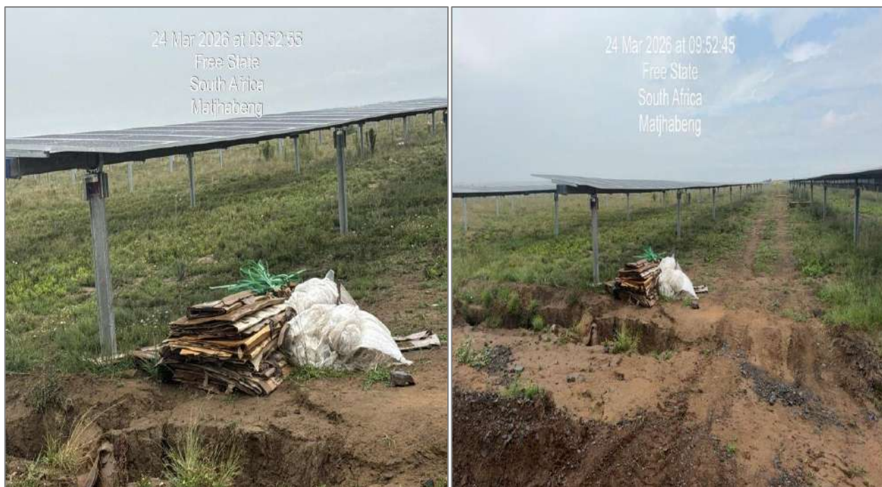
Figure 3: boxes on the solar field.
