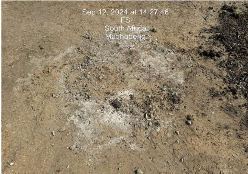
Figure 1: Concrete being mixed on the ground
