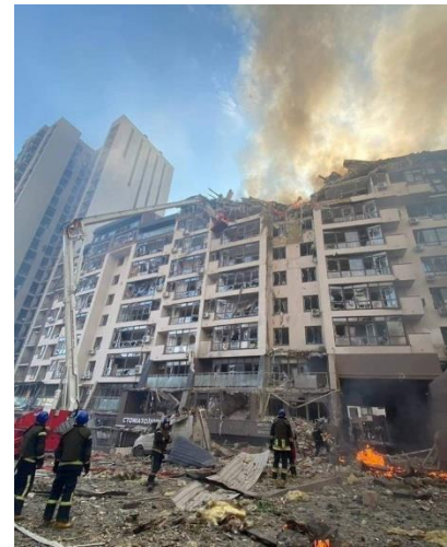
Residential building earlier today in Kyiv
