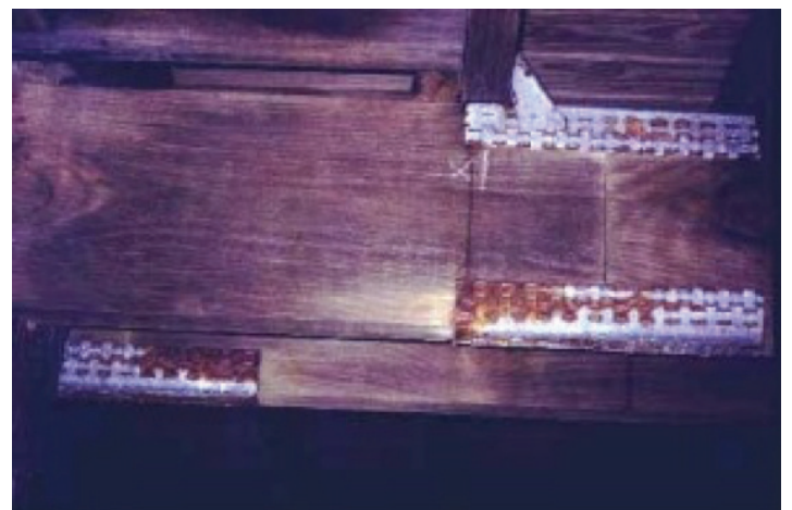
Photograph 2 - NOT ACCEPTABLE – Z275 connectors in deck joists 1 km from surf. 6 years old, Sunshine Coast.
