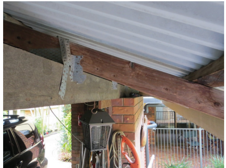
Photograph 1 - ACCEPTABLE – Z275 bracing, multigrips and truss plates in a Low Hazard (>10km from surf) Sheltered Condition. Note: Connectors have been installed for 35 years.
