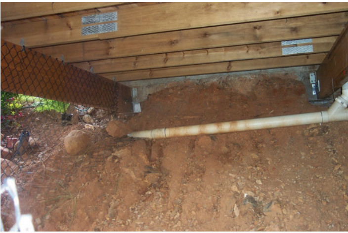
Photograph 3 - NOT ACCEPTABLE – Uncoated Z275 nail plates and framing anchors in Low Hazard Zone but Exposed Condition under a deck.
