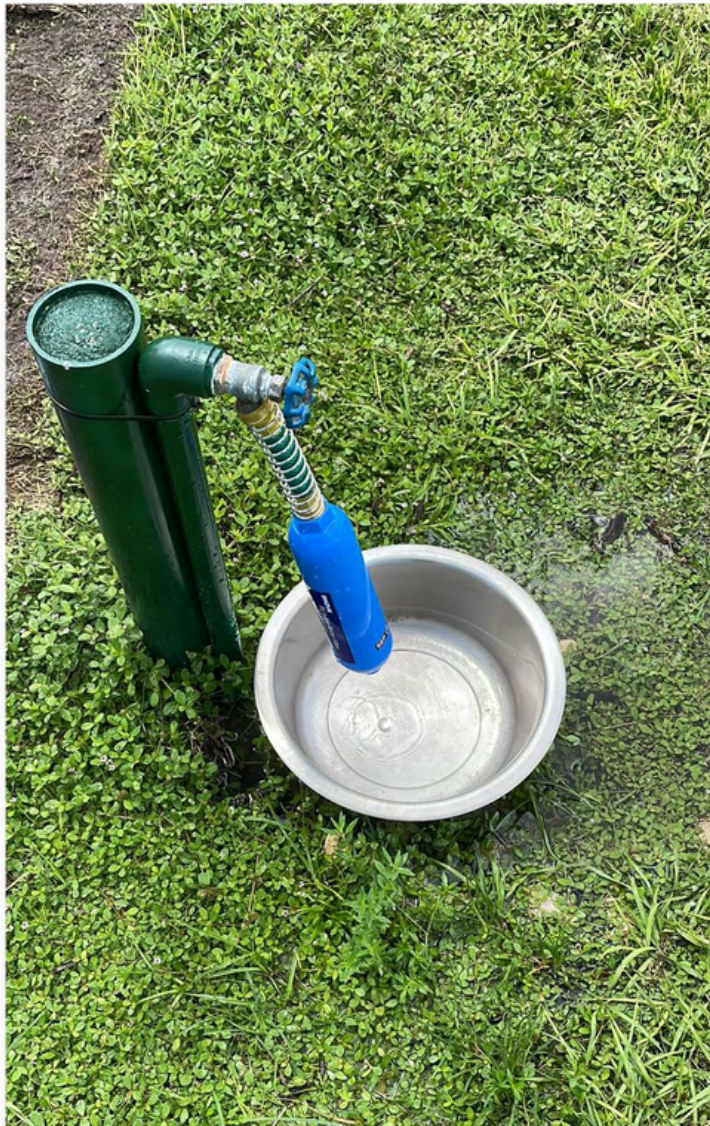
New water spicket and filter were installed at the dog parks.
