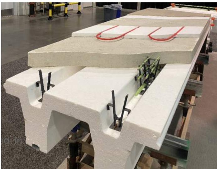
Figure 1 - Prototype of Climate Tech Building Systems Floor, Climate-Deck™
