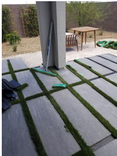
DSI LANDSCAPING – REAR YARD PAVER AND FAUX GRASS INSTALLATION
