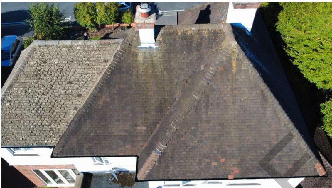
Original and extension roofs
