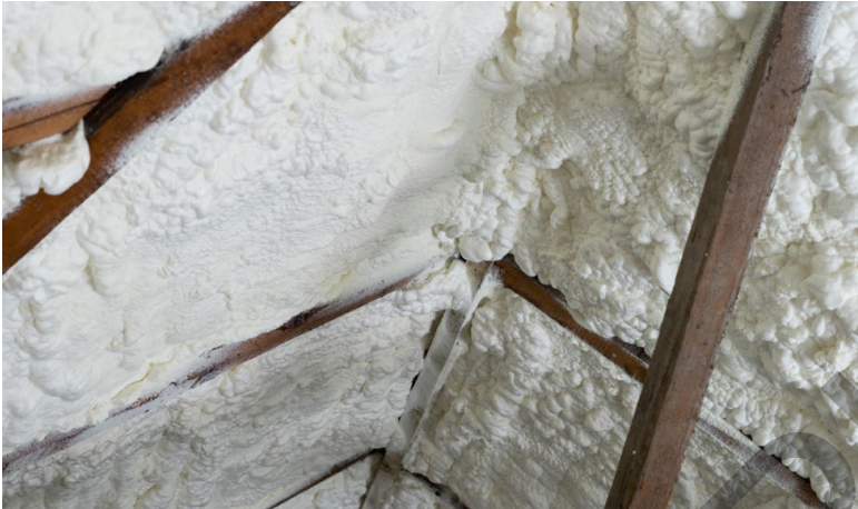
A typical sprayed foam installation in a roof space
