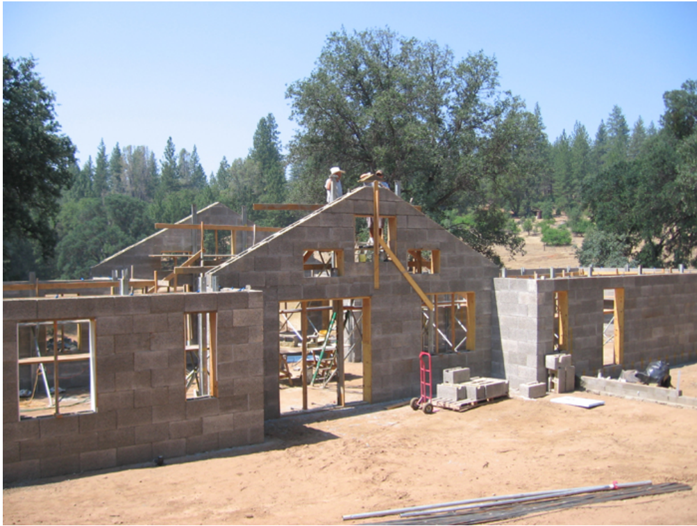
Passive Solar Durisol Home Under Construction.
