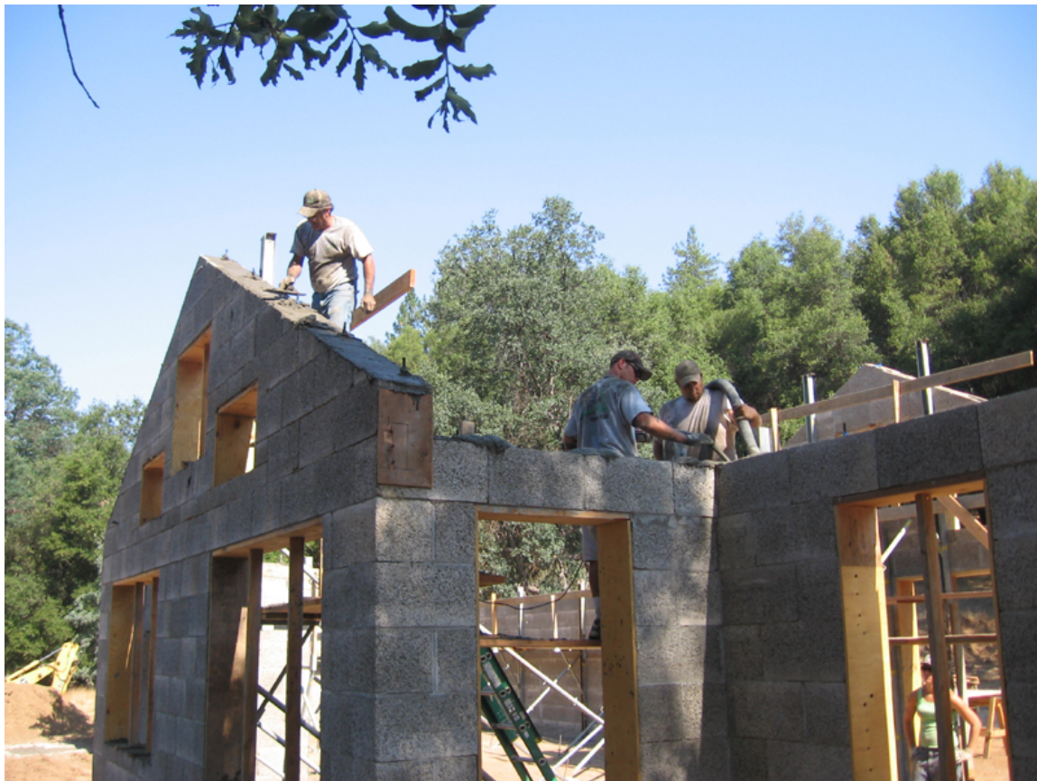
Filling the wall with concrete.
