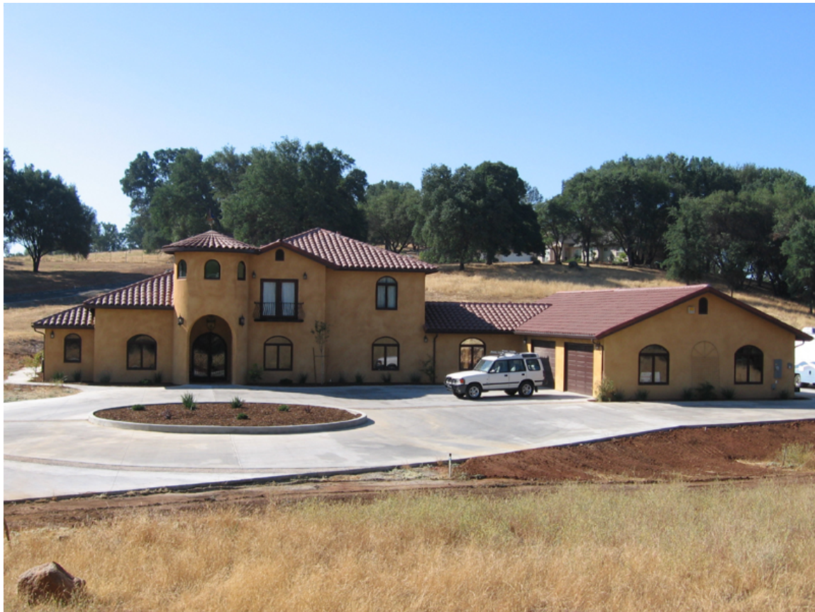
Custom home built by Hurst construction in Sonora California incorporating many state of the art features including a 5000 watt grid tie photovoltaic system, on demand water heater with a manifold plumbing system, radiant heat and super energy efficient windows and doors.
