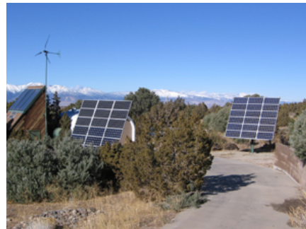
Two 1620 watt solar tracking arrays and a wind power power supplement make up the complete system. (Photo courtesy Sunfire research.)
