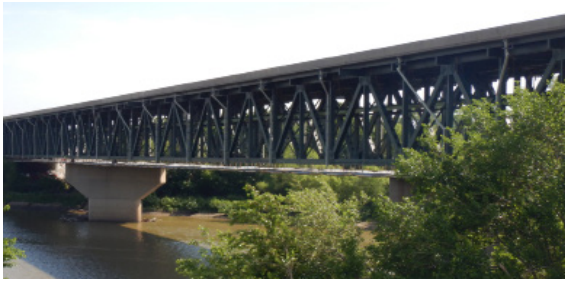
Above is an image of the 18th Street steel deck truss bridge.
