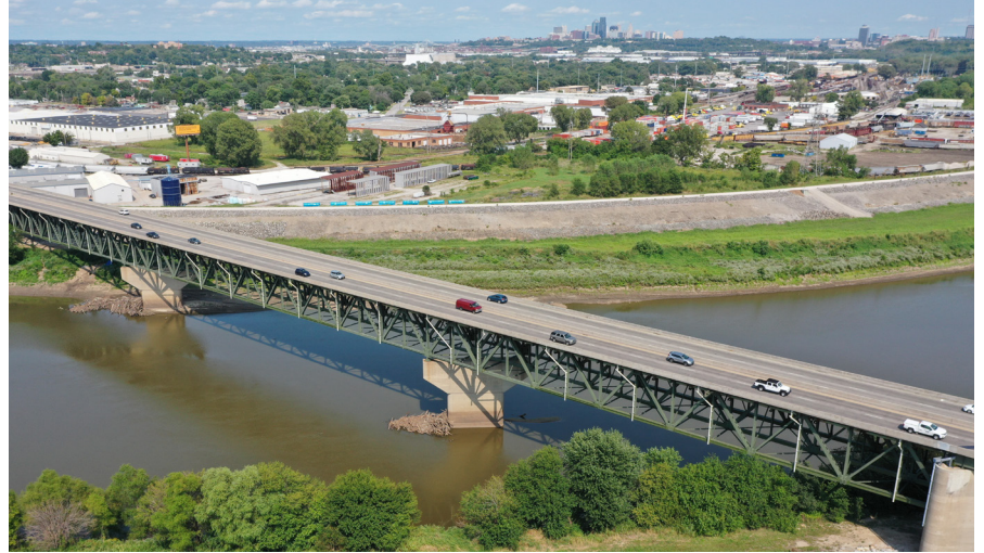
The 18th Street Bridge, built in 1959, is nearing the end of its service life.
