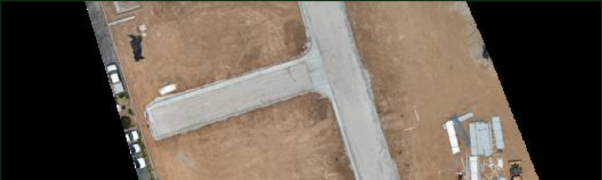
FOUNDATION / GRADING PROGRESS
