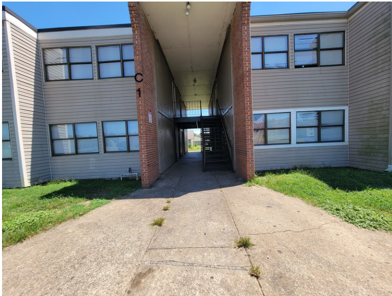
Picture #3: Apartment buildings
