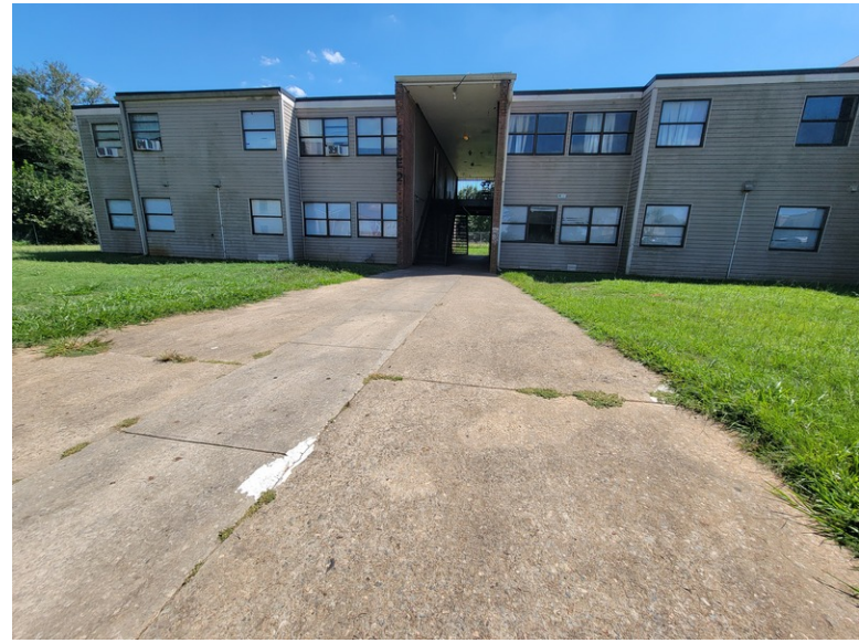
Picture #2: Paved walkway and apartment buildings
