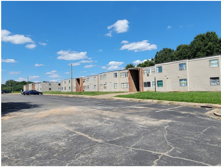
Picture #5: Parking areas and apartment building
