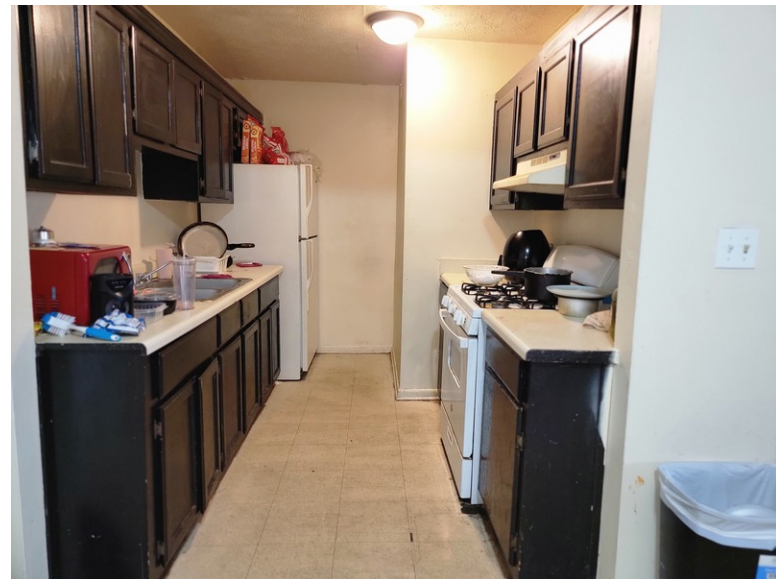
Picture #16: Non-friable vinyl floor tiles in an apartment
