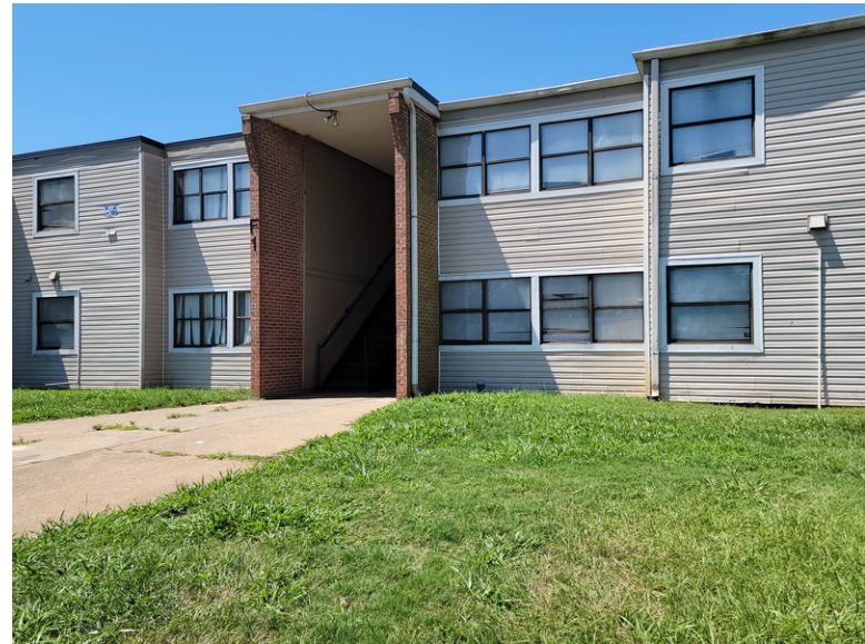
Picture #4: Apartment buildings
