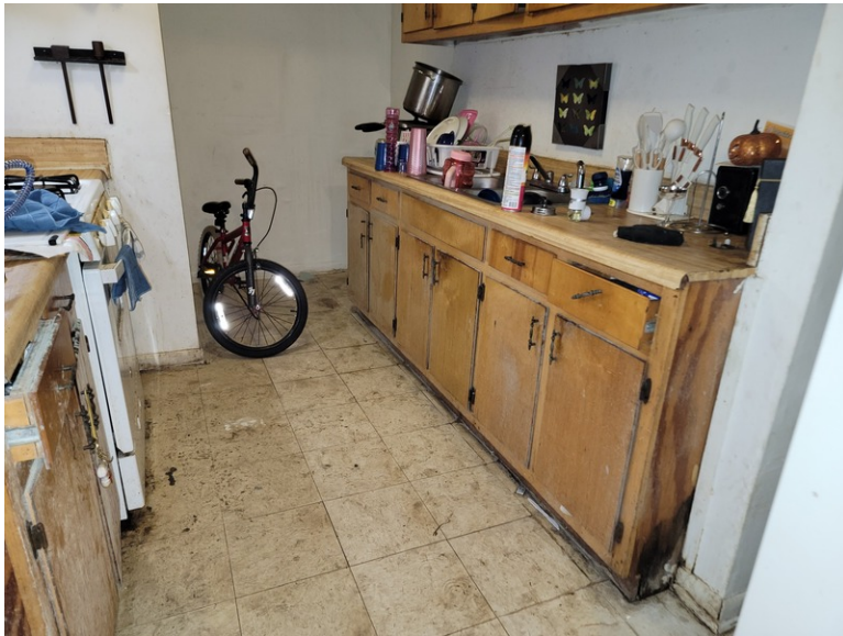
Picture #31: Apartment unit finishes
