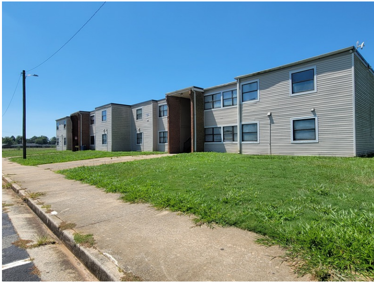
Picture #1: Apartment buildings
