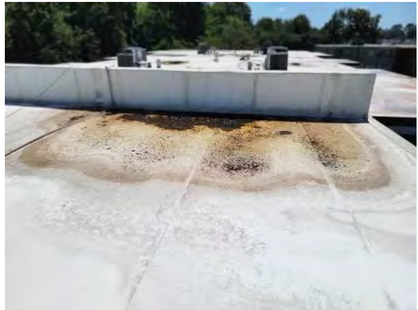
Picture #26: A typical roof
