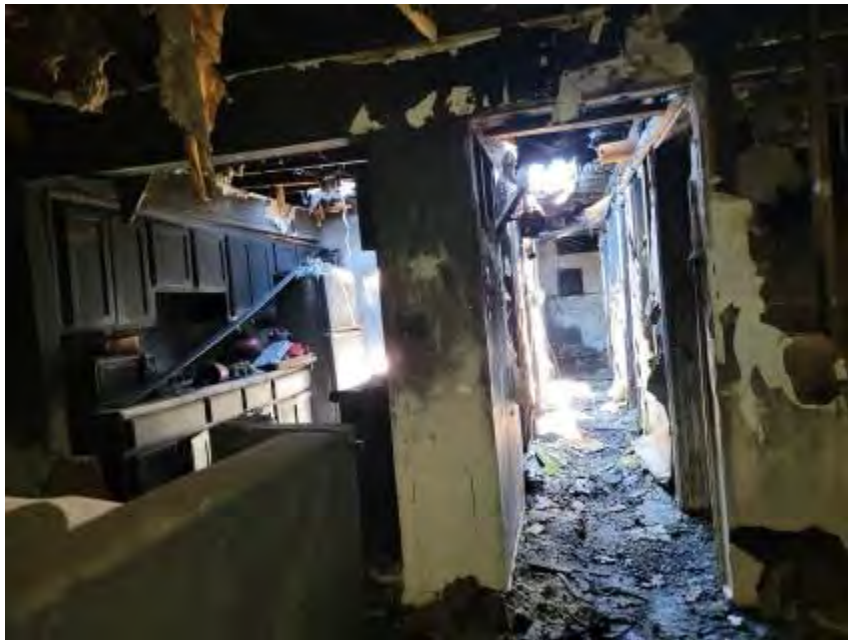
Picture #45: Unit C2-8
