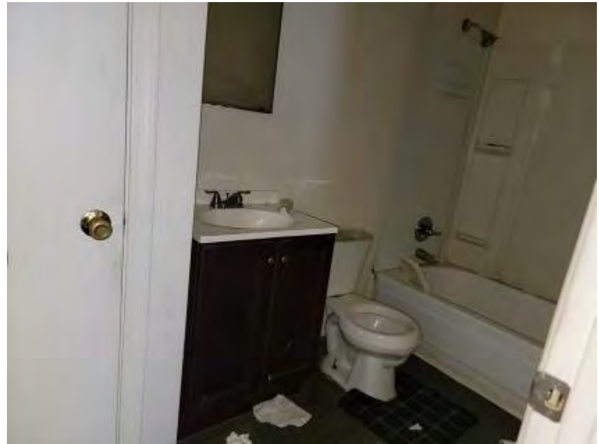
Picture #38: Typical bathroom finishes
