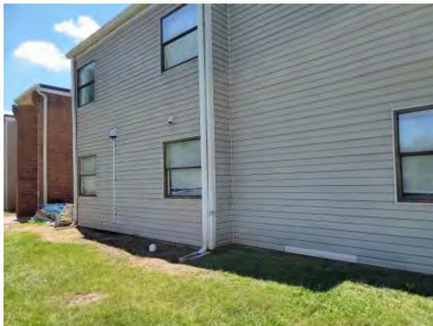
Picture #11: A typical building façade and gutter and leaders
