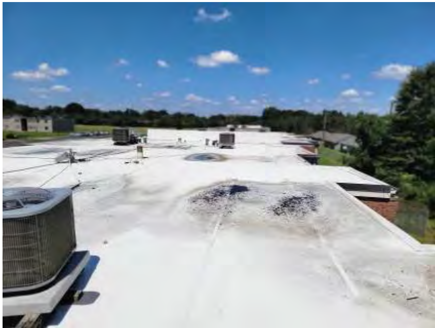
Picture #25: A typical roof
