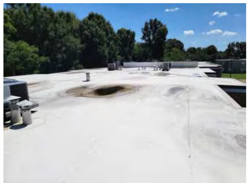
Picture #24: A typical roof
