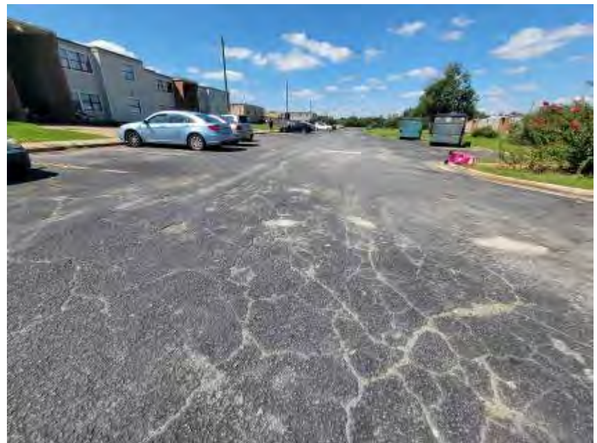
Picture #4: Asphalt-paved parking lot – note the trash dumpsters
