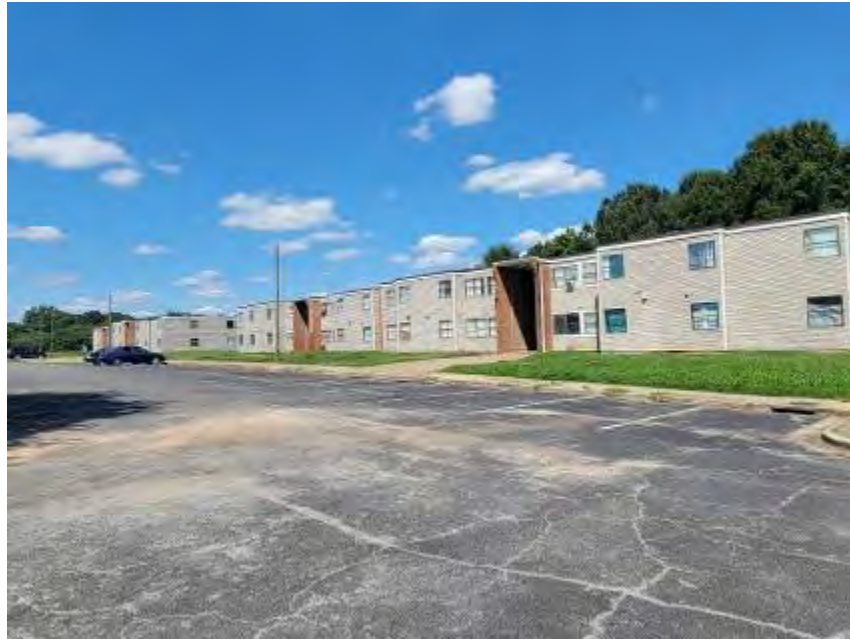
Picture #5: Asphalt-paved parking lot
