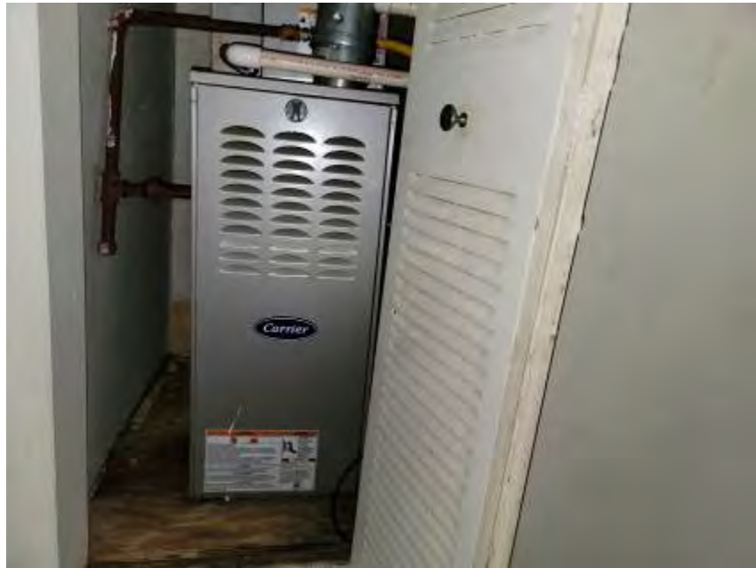
Picture #29: A typical furnace
