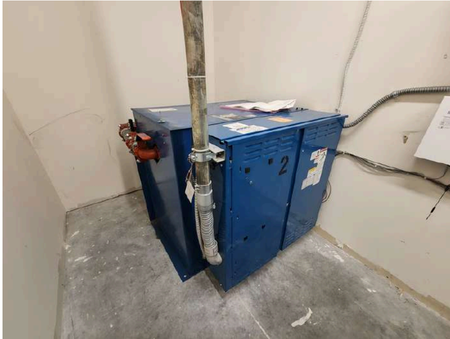
13. Elevator equipment at 8470
