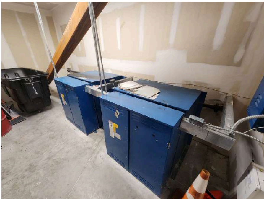
14. Elevator equipment at 8520
