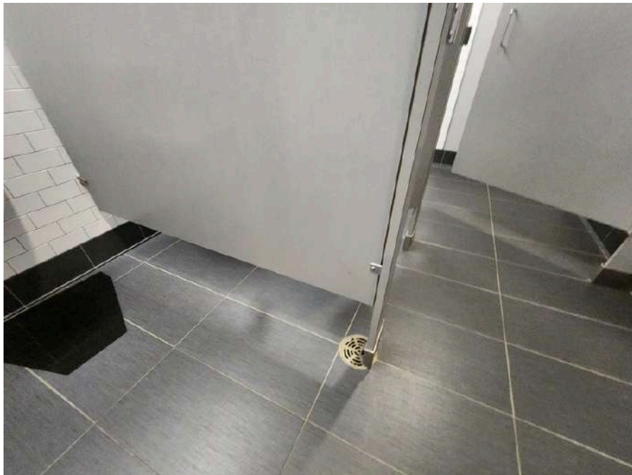
16. Floor drain in restroom
