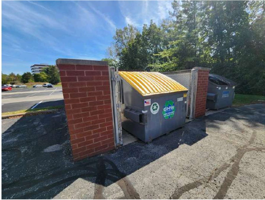
19. Dumpster enclosure at 8470
