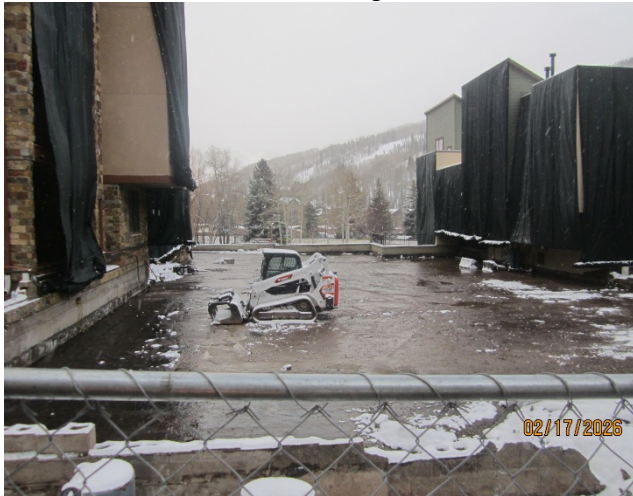
Overview / Looking South
