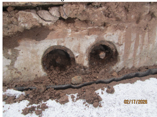
Existing PT Slab Cable Ends
