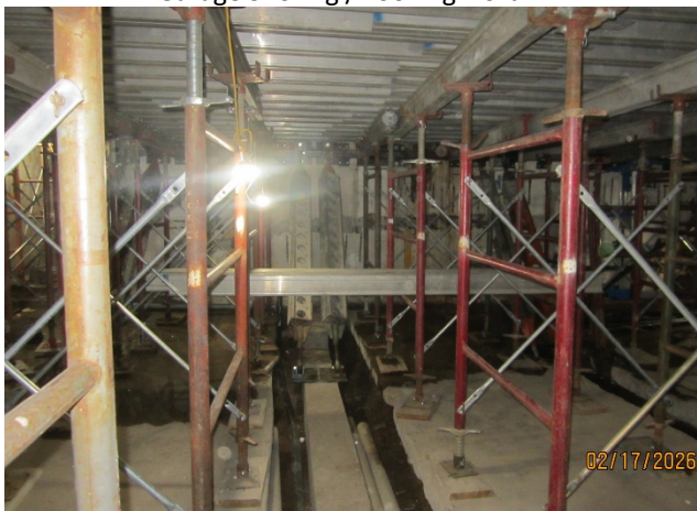
Garage Shoring / Looking North
