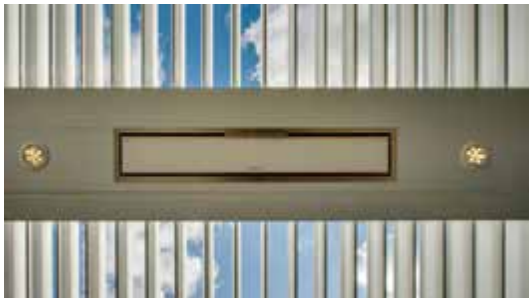
Beam Chases (Can Lights, Sonance Speakers etc.)
