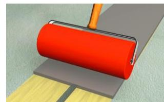
The sealing tape must be protected from mechanical damage. Therefore the edges of *HYDROFIX T* tape have to be covered with *HYDROPOX C* with a width of at least 50 mm.
