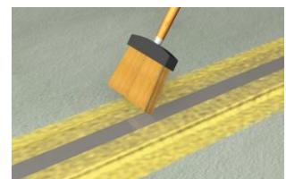
The longitudinal connection of tapes can be made by welding according to RVS 8T / DVS 2225-5 or by bonding with *HYDROPOX C* system adhesive. If welding grind the overlaps before with sandpaper (80 grit).
