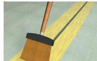
If it's dirty, *HYDROFIX T* tape is cleaned before by using a dry or wet towel (water, no solvent). After that the sealing tape is positioned on the adhesive layer during the open time of adhesive and rolled into the adhesive layer from the inside out with a wide draw roll. A full-surface bonding is necessary. Air pockets must be displaced outwardly by using the roll.
