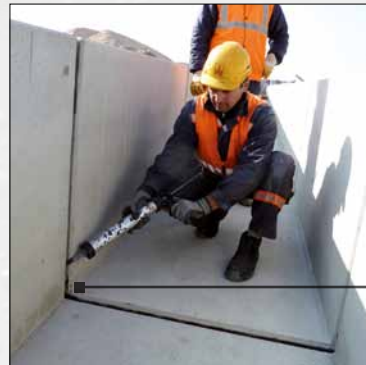
FIX-O-FLEX Kleb- und Dichtmasse Mastic adhesive and sealing compound
