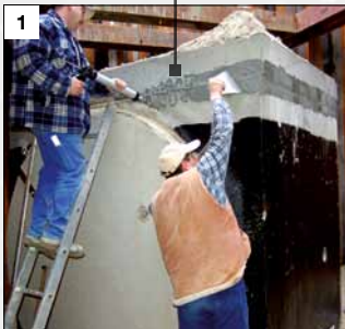
Schachtdeckelabdichtung in Braunschweig Manhole cover sealing in Braunschweig
