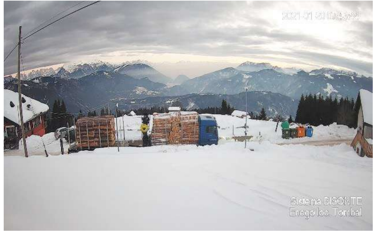
Enego: Installation at 1600m asl on the Alps
