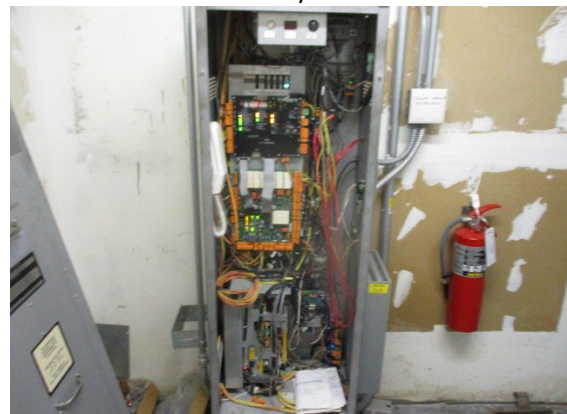
48 Elevator Control Board
