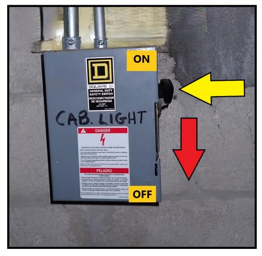
In addition to the large mainline power disconnect, there may be smaller disconnects with the same unique letter or number. The smaller disconnects are for the elevator cab lighting circuits and this disconnect should also be placed in the "OFF" position which ensures there is NO power going to the elevator cab during the weather event that could result in electronic component damage...
