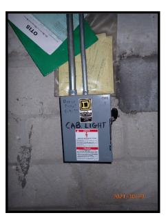
One (1) of the two (2) persons securing the elevator(s) should locate the elevator machine room(s), and the associated elevator mainline power disconnect switch(es). Each disconnect should be labled with a letter or numerical identification that is unique to each elevator which is very important to identify ensure the appropriate elevator is removed from service.....
