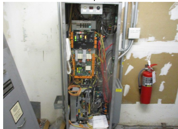
48 Elevator Control Board
