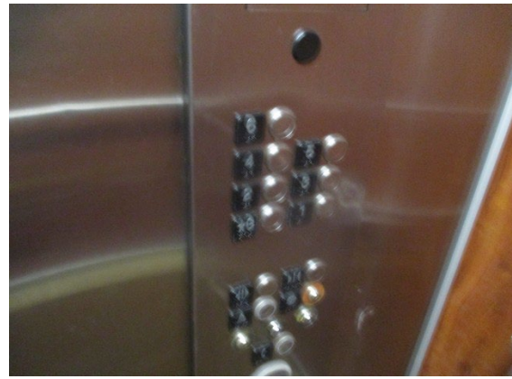
58 Elevator Cab Control Panel
