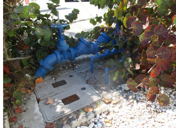
60 Backflow Preventor & Main Water Meters
