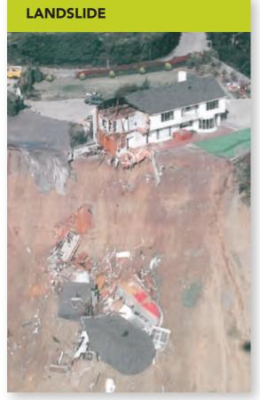
Earthquake shaking can be strong enough to cause soil and rock on a hillside to slide down the slope. A landslide can rip apart homes at the top of the slope and also crush homes at the bottom of the slope.
