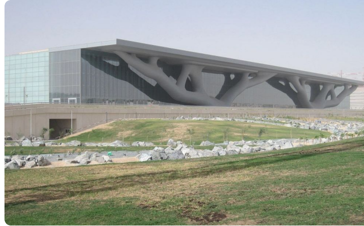
Qatar National Conference Centre Doha, Qatar:
