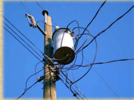
AC Power Pole
