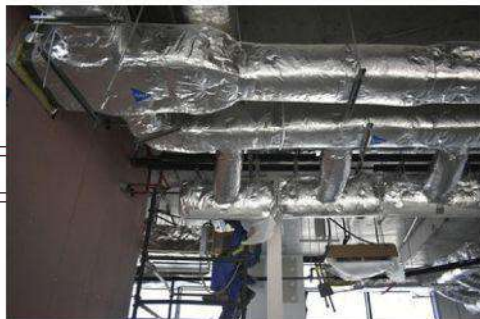
DUCT INSTALLATION
