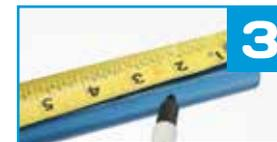
**Mark end of pipe** for the proper insertion depth
