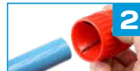
**Deburr** the end of the pipe outside and inside (a smooth edge allows easy fitting assembly and no damage to the fitting O-ring)
