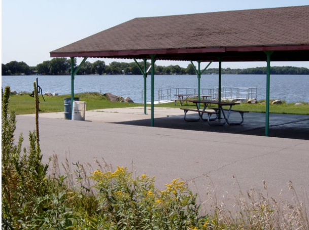
Photo: Picnic Shelter at King Mill Park. Taken by County Staff.
